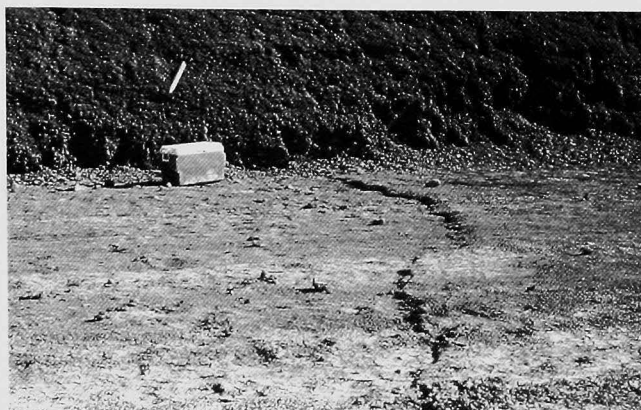
FIGURE 7: Asymmetrical heave feature in a graded cut caused by sudden, thrust-like heaving of the bedrock block on the right. This feature formed along a preexisting fracture plane. More than 30 cm of prior Holocene displacement was evident along the plane (at a point in the cut wall marked by the wooden stake) when the cut was first exposed. The heaving episode shown here occurred within 24 hr after a rainstorm and resulted in another 8 cm of total displacement.
