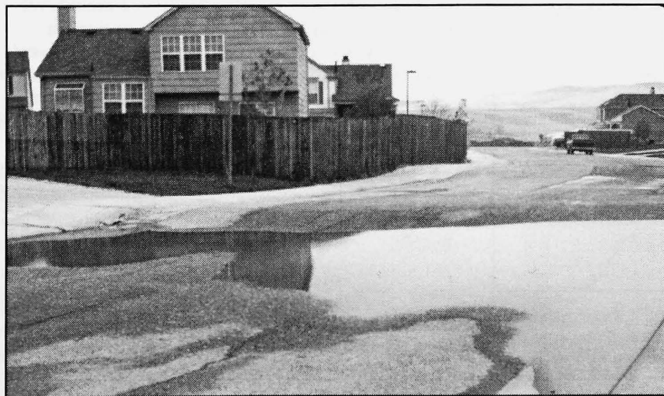
Figure 1. Linear heave feature associated with heaving bedrock in Douglas County. This heave feature has literally formed a dam that blocks storm drainage, resulting in surface-water ponding. Heaving bedrock has caused extensive damage in this neighborhood.
