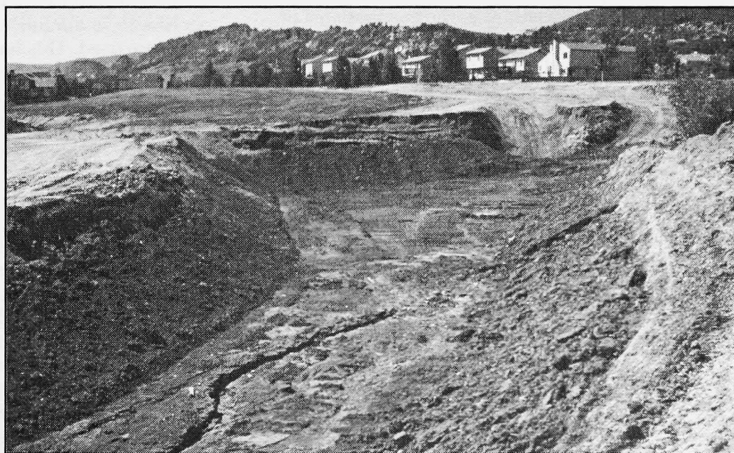
Figure 17. Overexcavation operation in progress at a subdivision in northwest Douglas County. The overexcavation area consists of a 16–20 foot deep cut that has been partially refilled with claystone as a sealant. The upper part of the cut was later filled with non-expansive material, and houses were built on the fill. beds are typically non-swelling.
