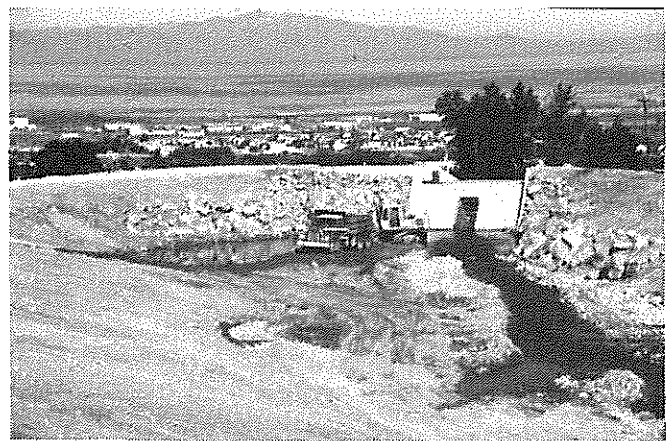
Figure 26. Rudd Creek debris basin in Farmington, Utah constructed in 1983–84 (photograph by Robert Kistner, Kistner and Associates).
