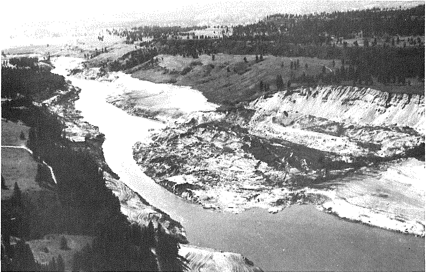
Figure 18. Jackson Springs landslide on the Spokane arm of Franklin D. Roosevelt Lake, Washington, 1969. This landslide was triggered by extreme drawdown of the lake (photograph by the U.S. Bureau of Reclamation).
