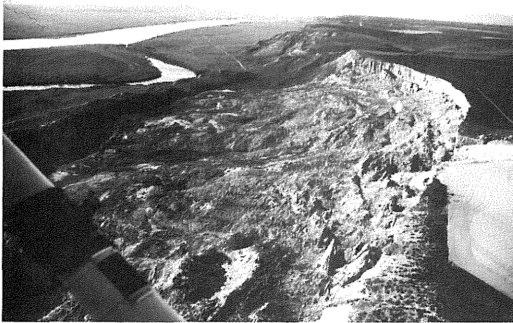
Figure 6. Aerial view of the Savage Island landslide on the east shore of the Columbia River, Washington, 1981. This landslide was caused by irrigation water (photograph by Robert L. Schuster, U.S. Geological Survey).
