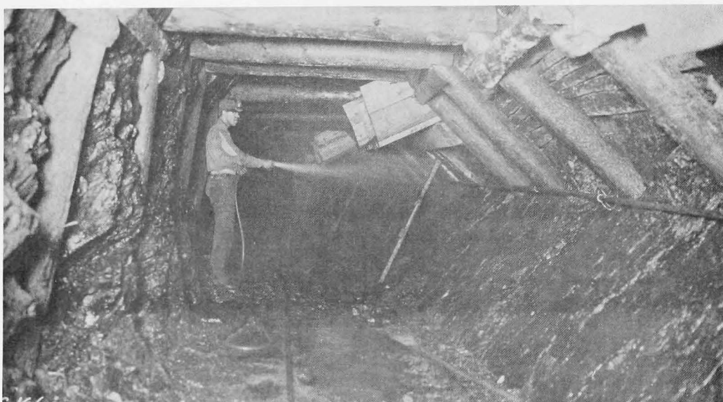
Figure 3. Coal chute into haulway in steeply pitching coal seam near New Castle (photo from Denver Public Library, Western History Department.)
