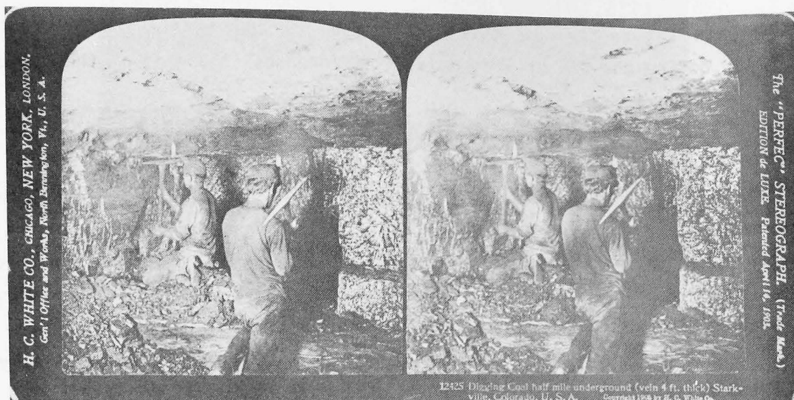
Figure 4. Stereoscopic photograph of pick mining at Starkville (photo courtesy Colorado Historical Society.)
