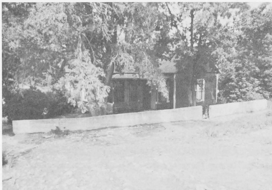
Figure 32. A, Deflection walls around houses near Portland Creek flume. B, Deflection wall around house near Cascade Creek flume.
