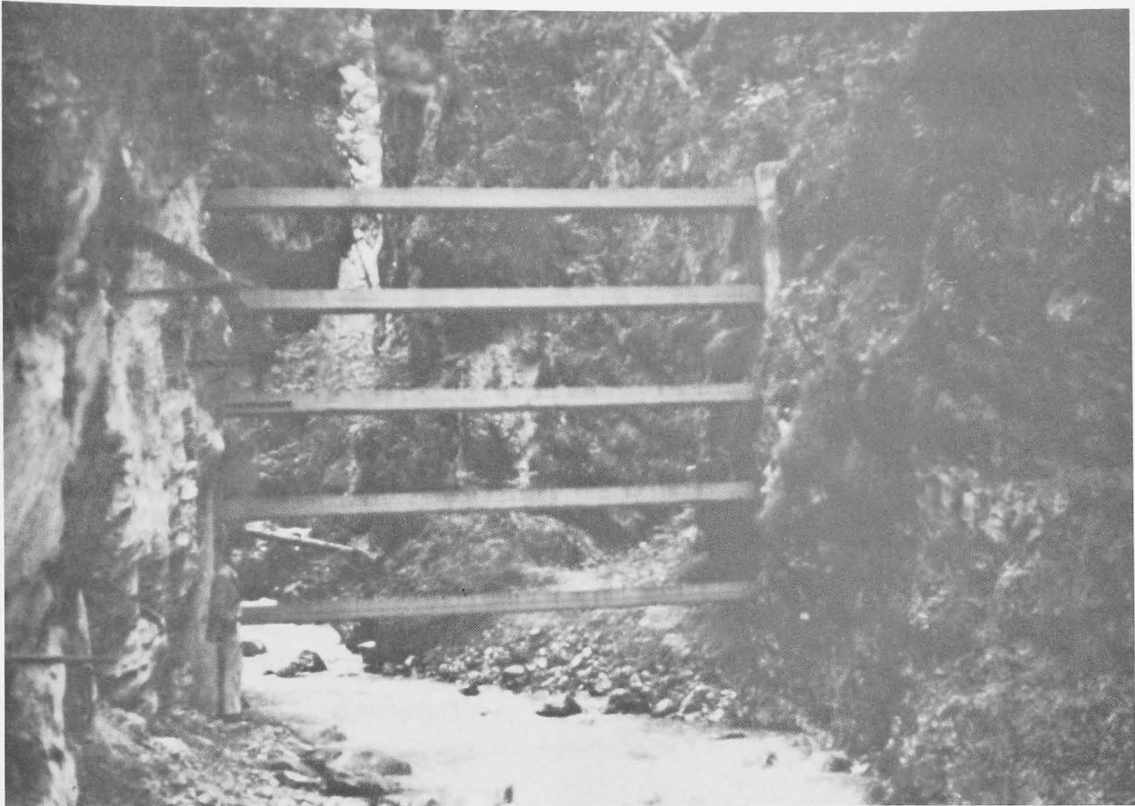
Figure 37. Debris fence. Example from Europe. (Photo courtesy Art Mears)
