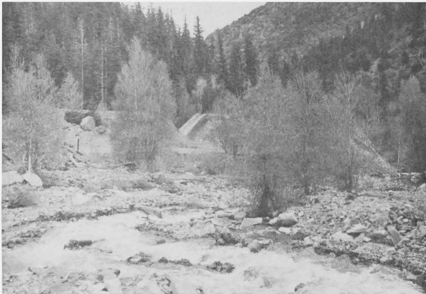
Figure 30. Mine tailings near the Bachelor Mine in Dexter Creek basin.
