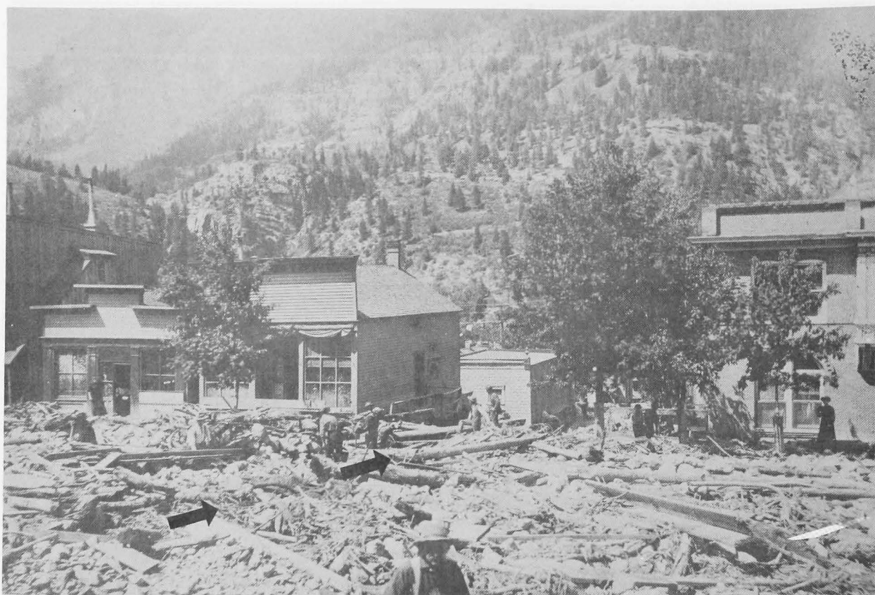
Figure 11. Debris flow on Portland Creek, 1909. Looking west across Main Street. Flume passes between buildings on left and tree (see arrows). (Photo courtesy Denver Public Library Western History Collection)
