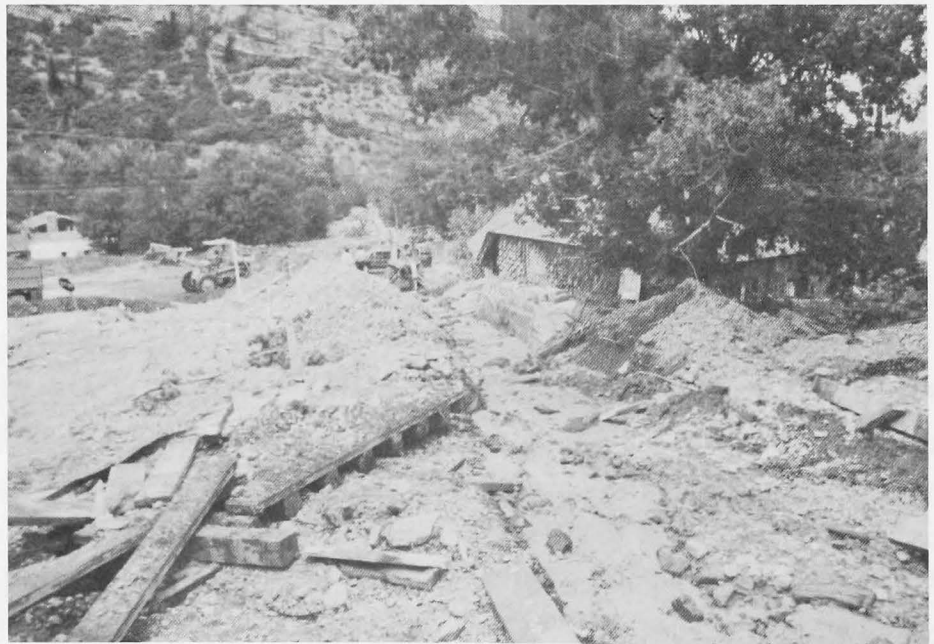
Figure 16. Debris back-up caused by plugged culvert on Cascade Creek at intersection with Highway 550, 1982 Looking west. (Photo courtesy William P. Stanton, CWCB)
