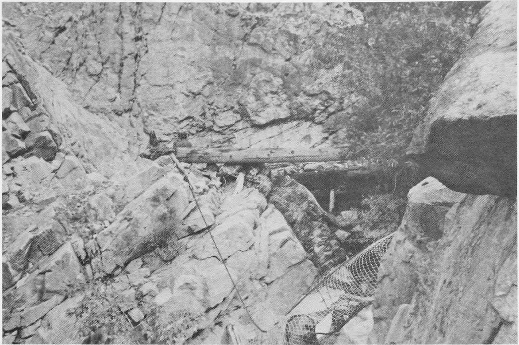
Figure 13. Remains of wooden diversion dam constructed on Skyrocket Creek in 1929. (Photo courtesy William P. Stanton, CWCB)
