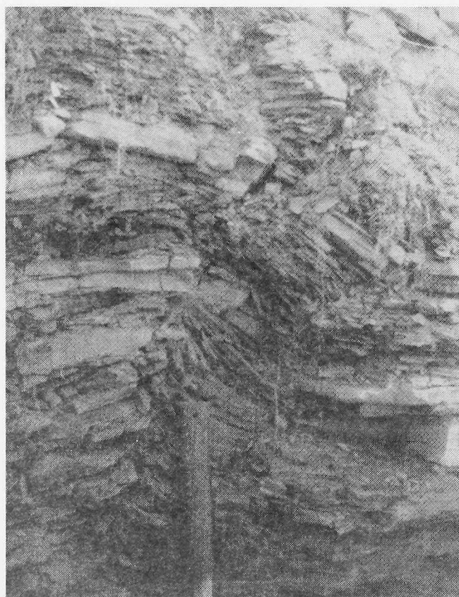
Fig. 4: Heave in the shale bedrock which is the foundation for the roadway. Heaving occurred due to concentration at the surface water by the roadway section.
