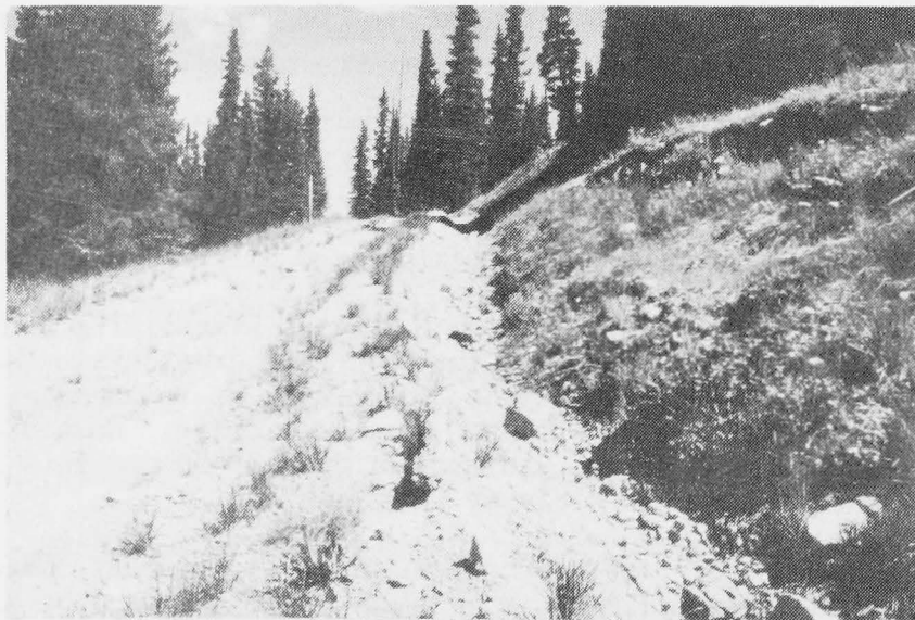
Figure 19. Crest drain on right above Borrow Area B. cut. Drain is effectively transmitting water through porous blanket although some sloughing has occurred.
