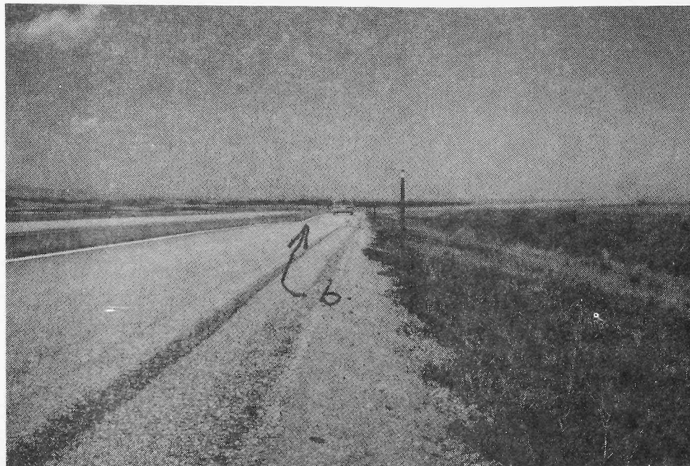
Fig. 3: Settlement failure due to collapsing soils derived from the tertiary shales. I-25 North Central Wyoming.
