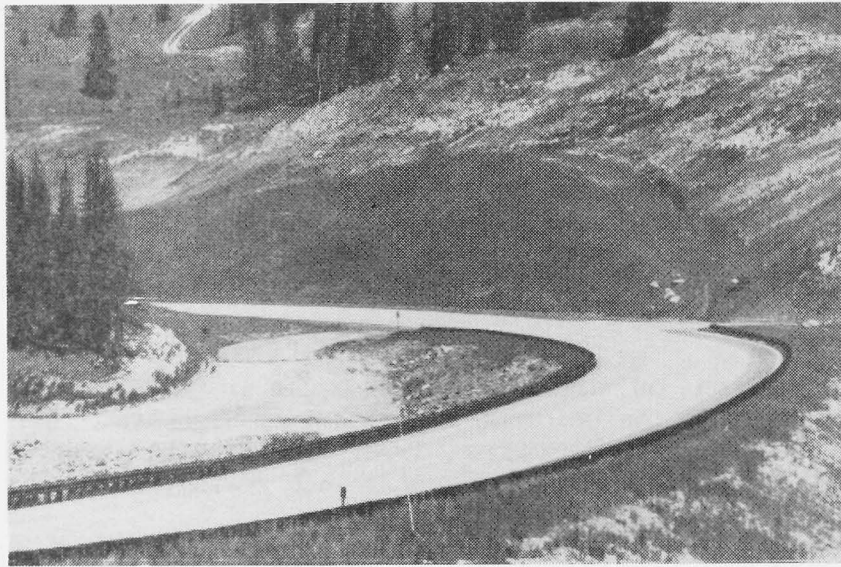
Figure 18. Borrow Area B. Berm (dark arcuate area) in lower part of cut has been an effective barrier to major failure.
