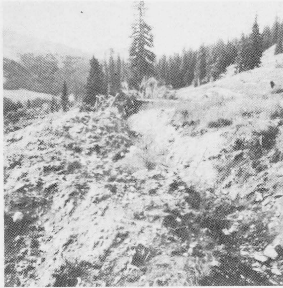
Figure 7. Glacial till exposed above Borrow Area B. Material on left (west) has slumped; note light-colored scar marking uphill limit of slump.
