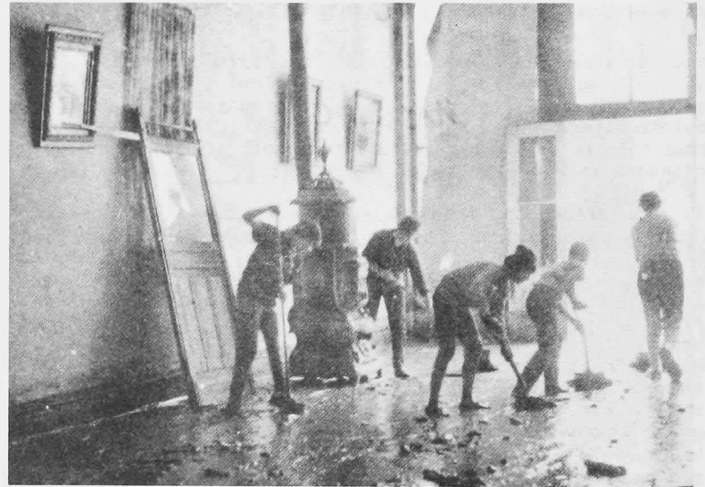
Citizens clean out the first floor of a building in Ouray after a flood early in this century.
