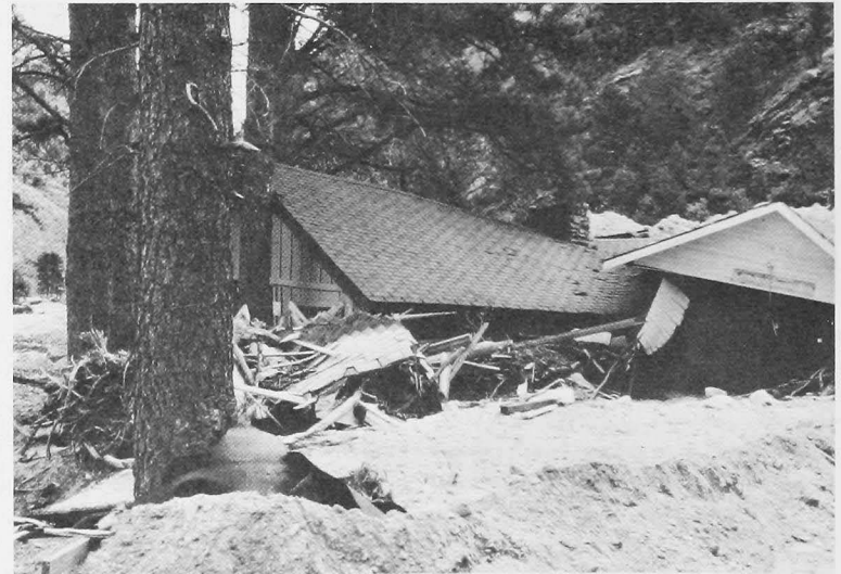
This house was totally destroyed by the 1976 Big Thompson flood. Note debris and sediment piled around the trees and the house.
