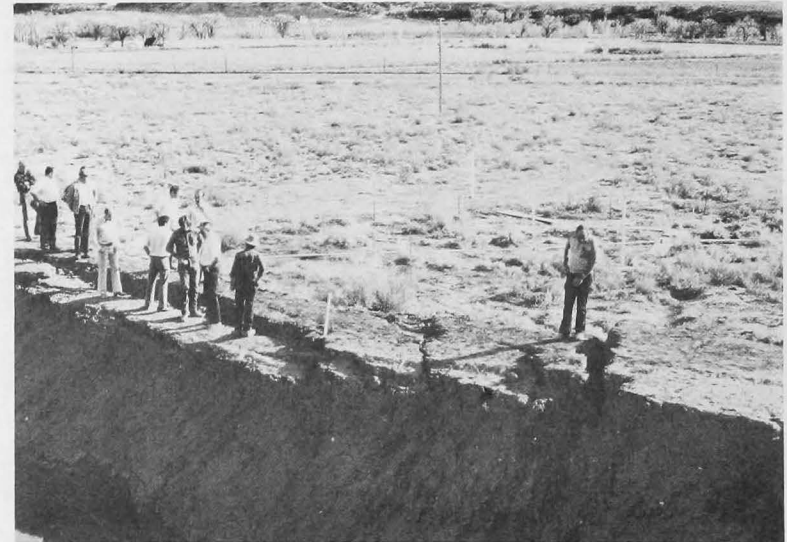
Tests permitted proper highway design and construction, avoiding future repairs.
