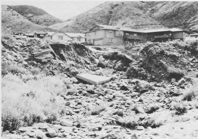
Housing development and drainage alterations caused this accelerated erosion near Golden.
