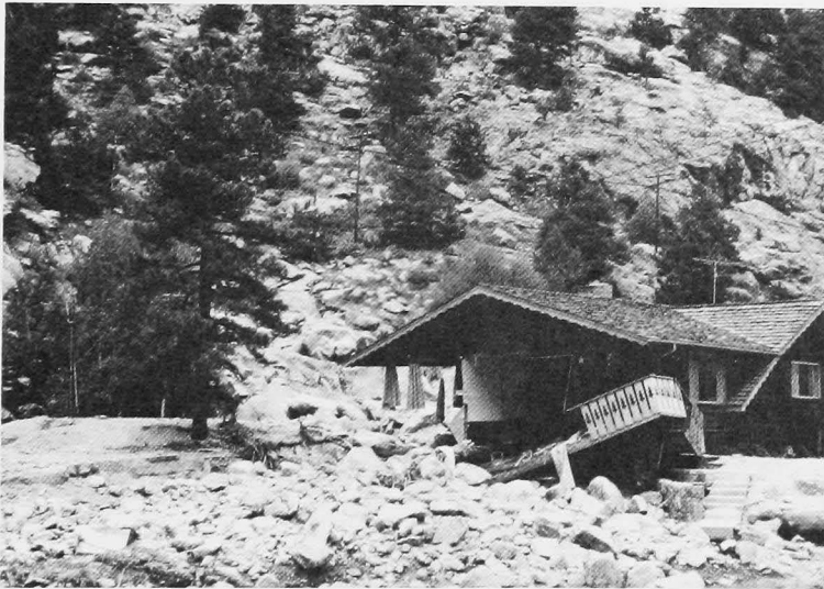
This house was located on a debris fan of a small tributary to the Big Thompson River. The house was not damaged by mainstream flooding on the Big Thompson, but by the debris flow from the small ravine behind the house.
