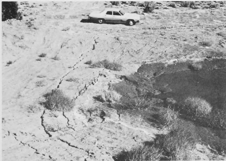
These two photos show hydrocompaction of soils along the proposed Interstate 70 alignment near Rifle. Note concentric rings around the pond and through a test road embankment.
