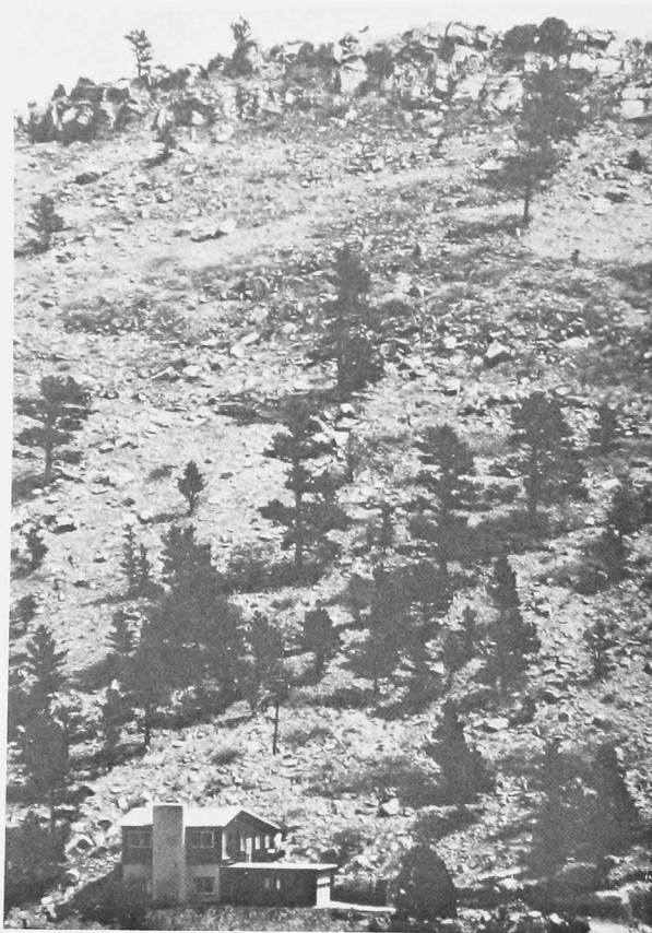
Figure 13. ROCKFALLS ARE COMMON IN AREAS LIKE THIS. NOTE THE NUMEROUS RANDOMLY ORIENTED LARGE BLOCKS OF ROCK ALL OF WHICH WERE DERIVED FROM THE CLIFFS ABOVE. ROCKFALLS ARE UNPREDICTABLE IN TIME AND EXACT LOCATION, AND IN AREAS LIKE THIS PERMANENT HUMAN HABITATION IS ALMOST ALWAYS UNSAFE.
