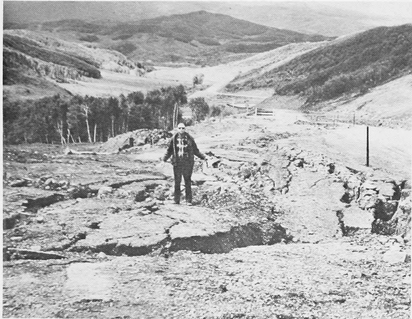
Figure 11. THIS HIGHWAY, BUILT IN A HIGHLY UNSTABLE AREA, WAS SEVERELY DAMAGED BY A LANDSLIDE.
