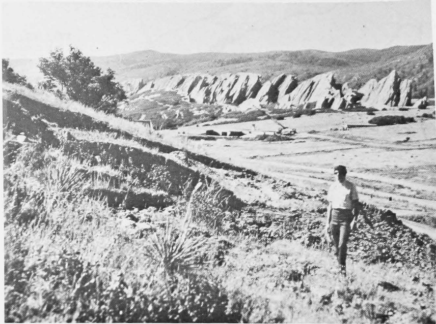
Figure 9. A SMALL LANDSLIDE THAT WAS INITIATED BY A ROADCUT SHOWS SEVERE GROUND BREAKUP. RESIDENTIAL DEVELOPMENT WAS CONTEMPLATED IN THIS AREA.
