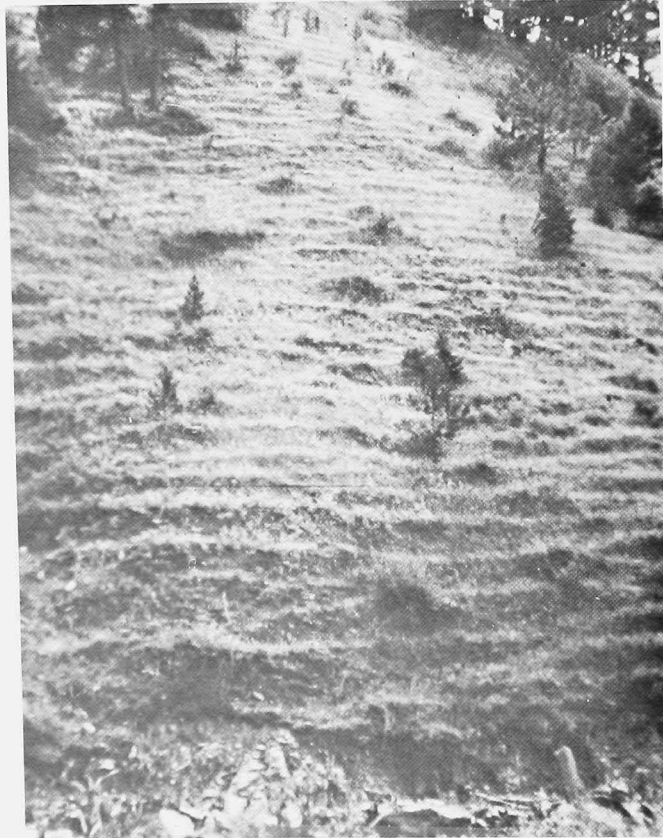
Figure 21. ACCELERATED DOWNHILL CREEP OF SURFICIAL MATERIALS MAY RESULT IN SOIL RIPPLES SUCH AS THESE. THIS TYPE OF SLOPE MOVEMENT CAN BE DESTRUCTIVE TO MANY KINDS OF CONSTRUCTION IF IT IS NOT RECOGNIZED OR IF STRUCTURES ARE IMPROPERLY DESIGNED.
