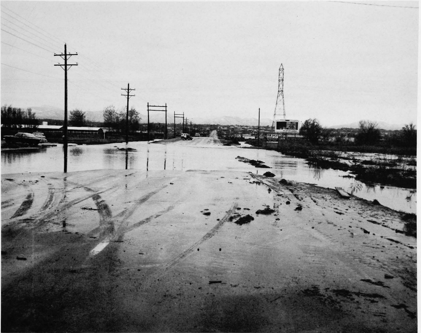
Figure 4. Flood damage on State Highway as result of thundershower in foothills region.
