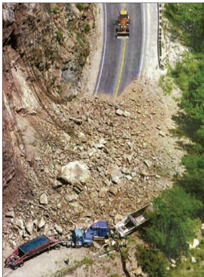
Figure G: Aerial view of the Clear Creek Canyon rockslide. Note how fallen rock pushed the blue and white haul truck across the roadway to hit, head on, with another haul truck (blue and red). Luckily the blue and white truck was not buried and crushed in the debris. Draped wire mesh shown hanging from the outcrop (upper left of photo) was not designed for such a massive rockslide. (Photo courtesy of the Denver Post.)
