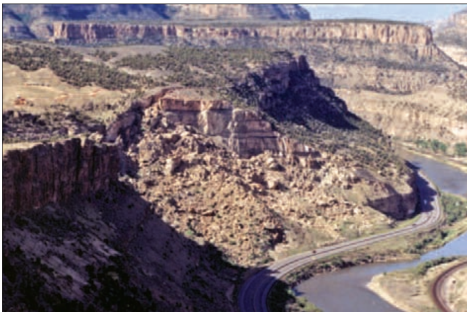
Figure C: Oblique view of the DeBeque Canyon rockslide. Note the large blocks in the rubble and how the river course has been diverted and narrowed. The ground fissure can be seen at the headwall of the landslide, left of center. Interstate 70 crosses the toe of the landslide. (Photo by Jon White.)
