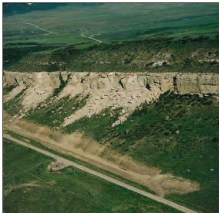
Figure J: Subsidence of the Foidel Creek Mine resulted in rockfall in the Twentymile Sandstone cliff face. Note rockfall ditch and berm above roadway. (Photo courtesy of Colorado Division of Reclamation, Mining, and Safety.)
