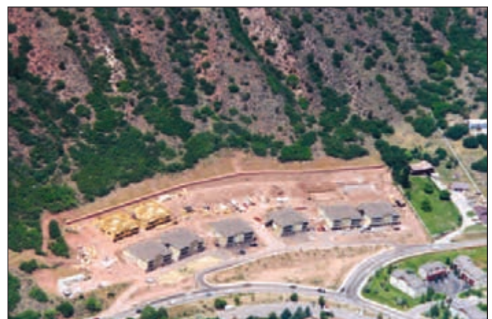
Figure C: This newer development in west Glenwood Springs constructed a rockfall impact wall above their townhomes to protect against both rockfall and mudslides (debris flows). (Photo by Jon White.)
