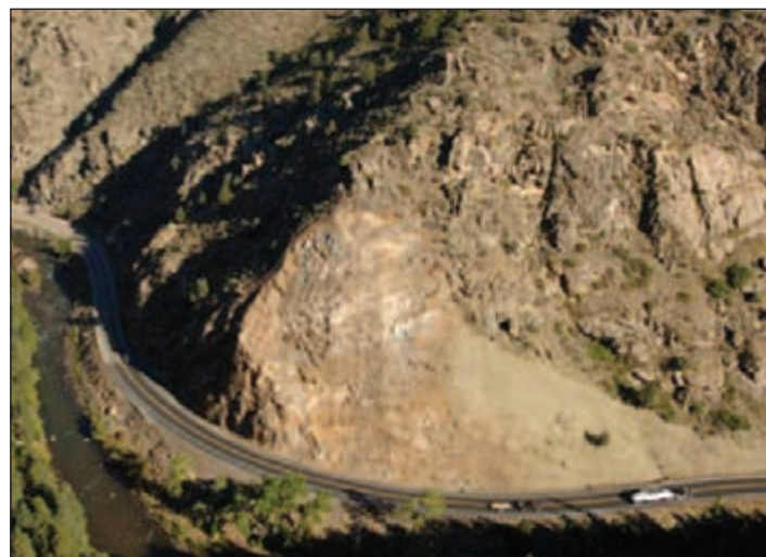
Figure I: Oblique aerial photo of rockslide area after rock excavation project. (Photo by CDOT.)
