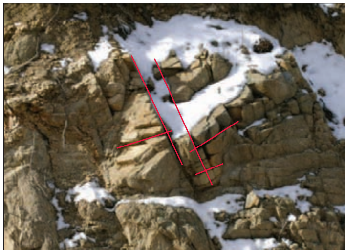
Figure 3: Discontinuities (cracks and fractures, some shown with red lines) in a Precambrian gneiss outcrop near Evergreen, CO. Weathering processes continually work to break apart the rock mass. The fractures are obvious zones of weakness. The orientation of the fractures is important in assessing rockfall hazard. (Photo by TC Wait)
