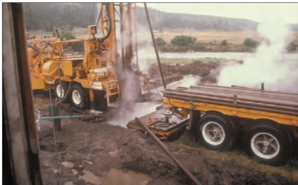
Drilling to evaluate the geothermal potential at Poncha Springs, Chaffee County. Potential is recognized by measurement of high heat flow on the surface and drilling is carried out to test the temperature of waters at depth. Photo by Jim Cappa.
