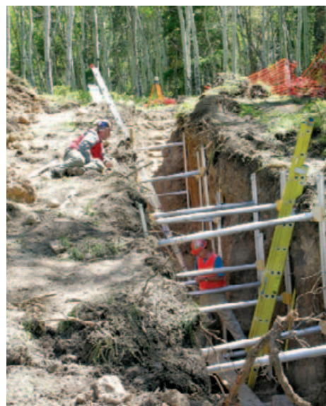
Trench excavated by CGS through the Williams Fork Mountain Fault in Grand County
