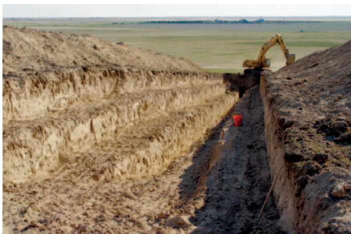
Anton trench excavated by CGS in Washington County
