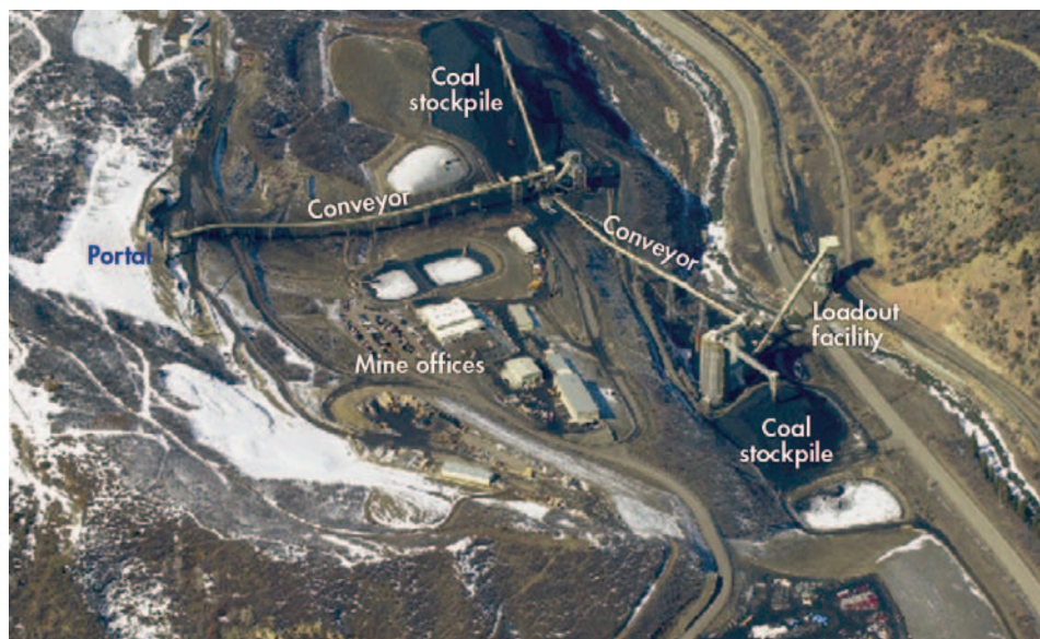
Figure 14. Aerial view of the Arch Coal West Elk Mine, Gunnison County, Colorado. Visible on the surface are the long conveyor lines between the portal and the coal loadout facility. Photo courtesy of W. Koontz, West Elk Mine.
