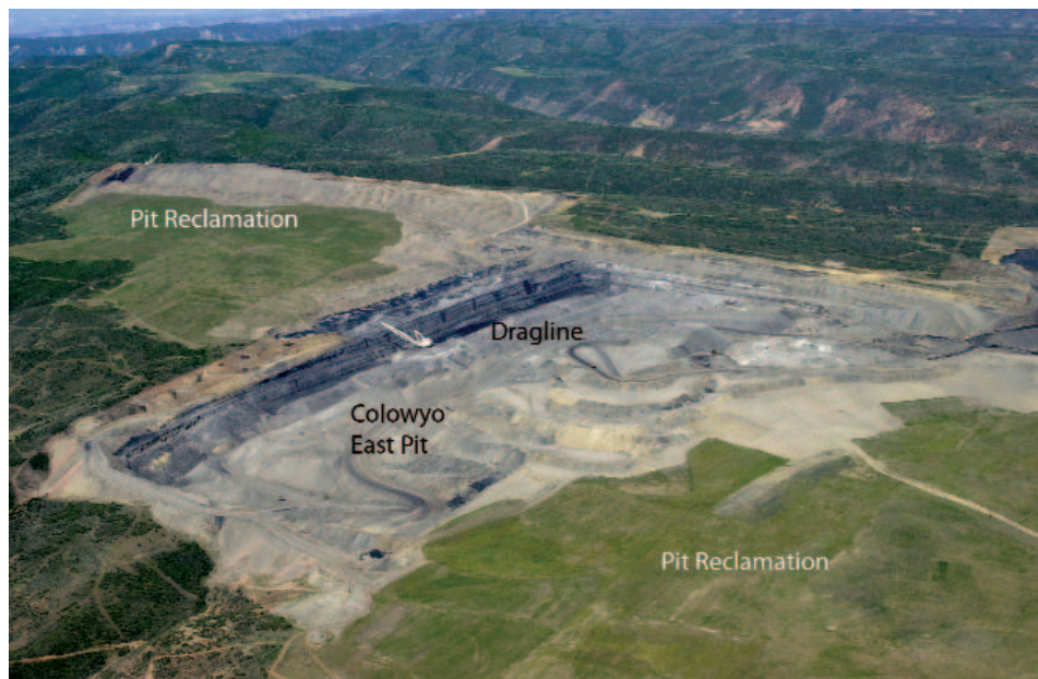
Figure 13. Oblique aerial view of active surface operations at Kennecott's Colowyo coal mine, Moffat County, Colorado. Note the draglines for scale. Reclamation occurs simultaneously as the pit advances. Photo courtesy of D. Berry.
