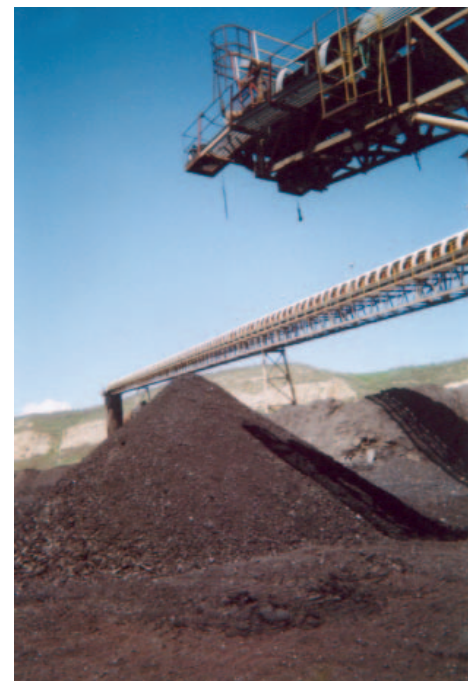
Figure 8. Coal conveyors at the Peabody Energy Company’s Twentymile/Foidel Creek Mine, Routt County.
