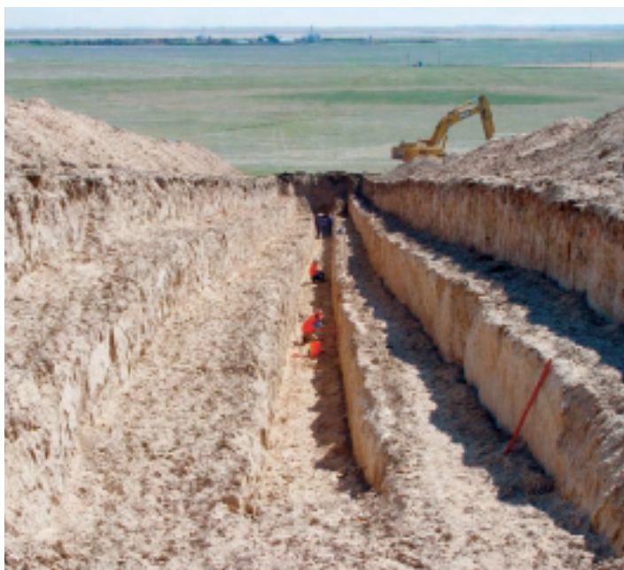
Geologists logging the 15-foot deep, 600-foot trench
