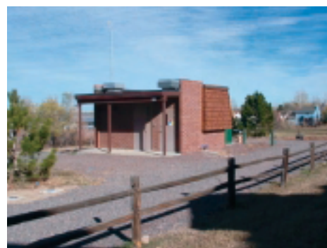
Denver Basin Aquifer Recharge Demonstration Project well house near Highlands Ranch. Wells used for groundwater recharge can be installed wherever the best aquifer conditions occur because of their small area of disturbance—even in the midst of a subdivision.
