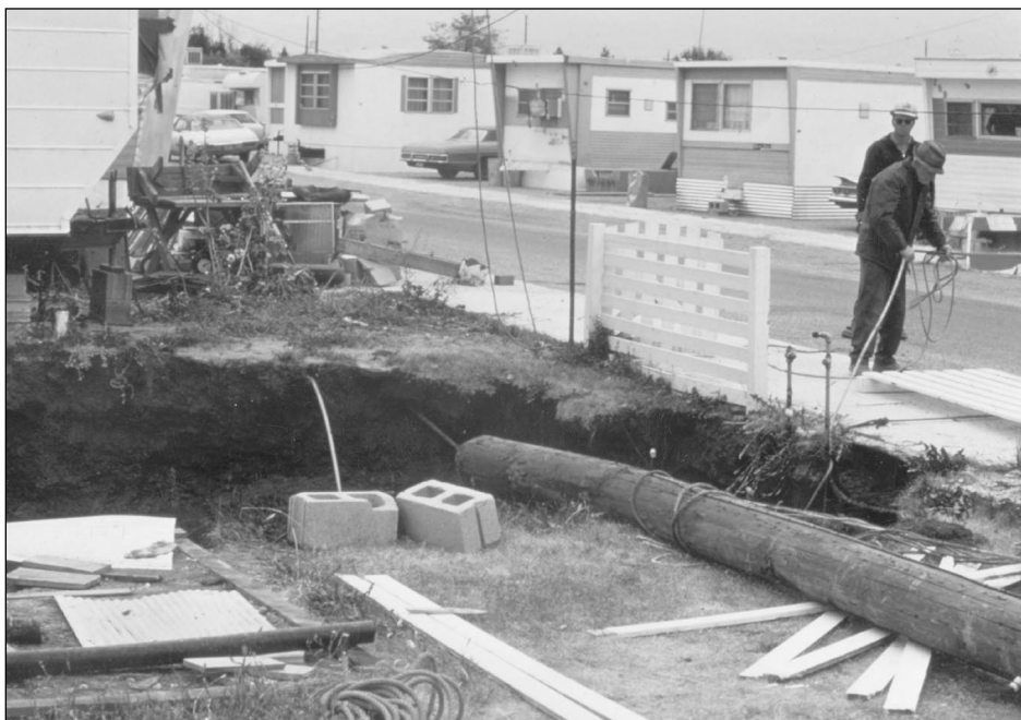
Coal mine shaft collapse in a trailer park in Colorado
