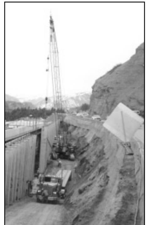
Retaining walls at Highway 82 Shale Bluffs project PHOTO BY R. PIHL
