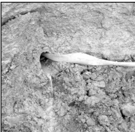
Close-up of a completed wick drain installation (State Highway 13)
