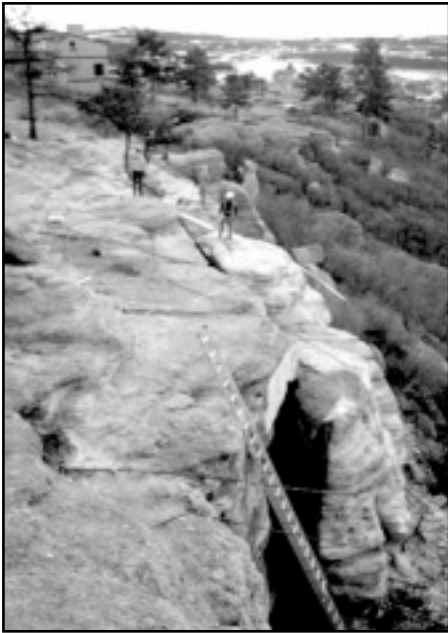
Castle Rock: remedial work at top of rock
