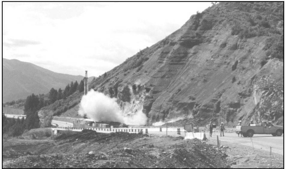
Blasting Highway 82 re-alignment at Shale Bluffs PHOTO BY R. PIHL
