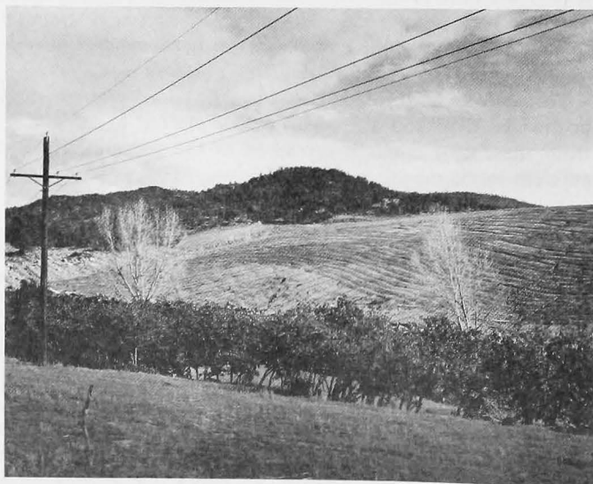
Figure 6. View to northeast across York Canyon showing mined-out areas that have been graded and covered with topsoil.
