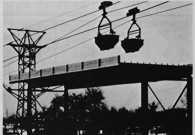
Figure 11. Bicable tram at limestone quarry and cement plant in West Germany.
