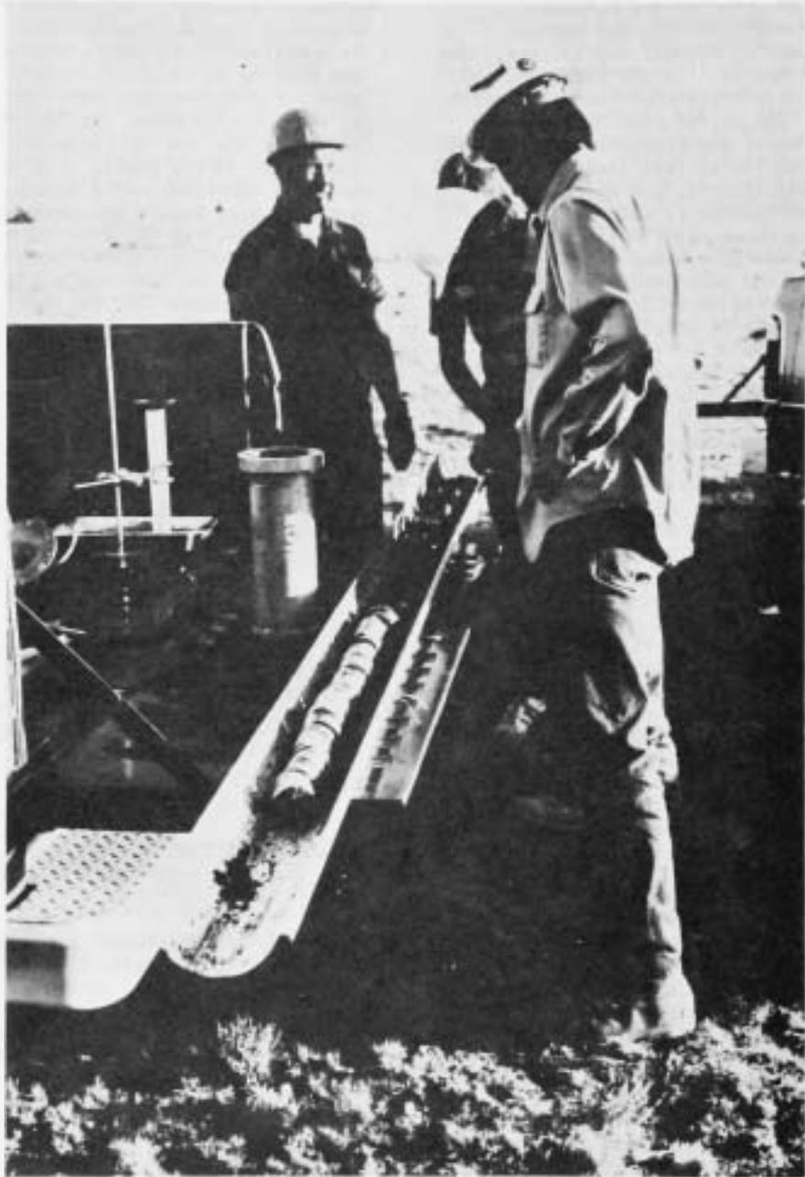
Laying out core preparatory to placing coal in methane desorption cylinder, Huerfano County, Colorado
