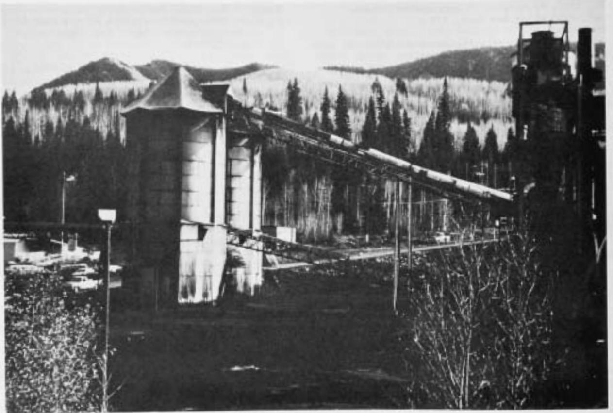
Tipples and thermal dryer, underground coal mine, Coal Basin, Pitkin County, Colorado
