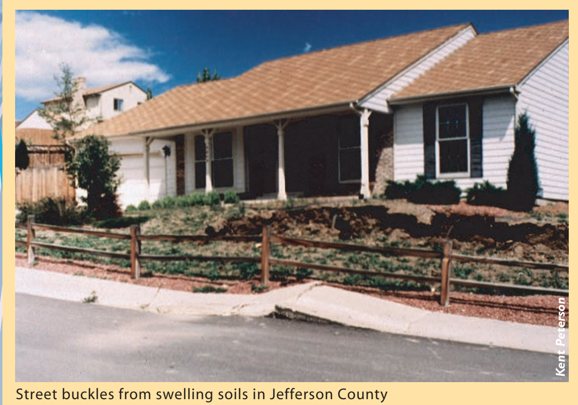
Street buckles from swelling soils in Jefferson County
