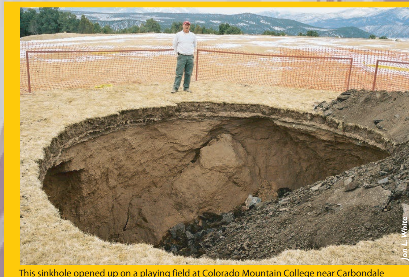
This sinkhole opened up on a playing field at Colorado Mountain College near Carbondale
