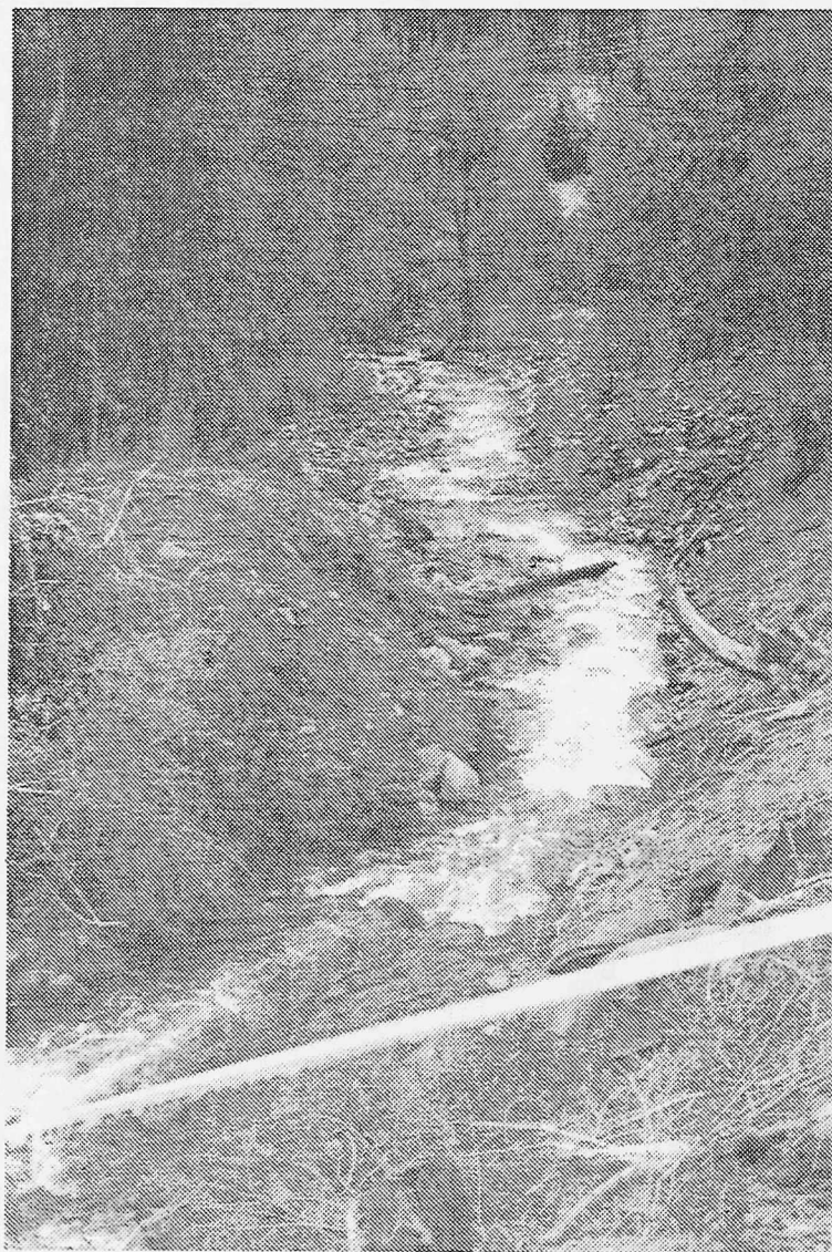
Figure 3. Location of whirlpool and cribbing encountered during re-alignment of Silver Creek Channel. The loose fill material on the left side of the creek in the center of the picture was dumped into the whirlpool.
