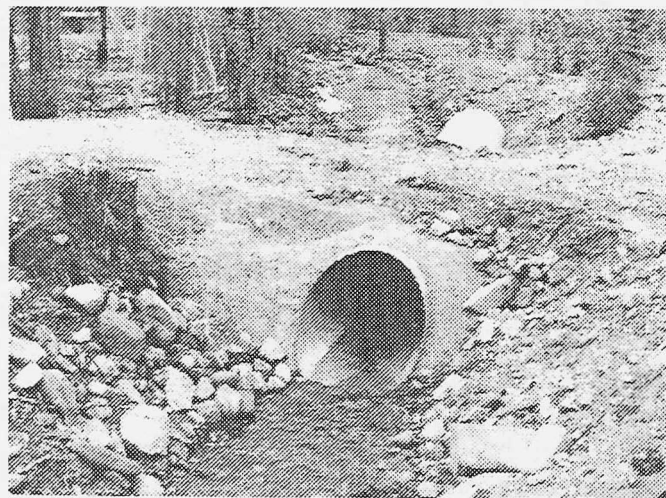
Figure 9. Silver Creek culvert over caved-in area of Atlantic Cable Mine.
