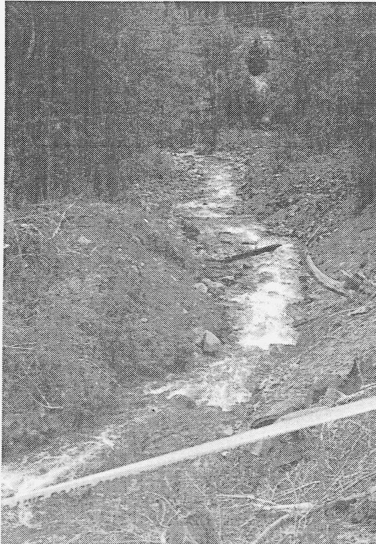
Figure 4. Location of whirlpool and cribbing encountered during re-alignment of Silver Creek channel. The loose fill material on the left side of the Creek in the center of the picture was dumped into the whirlpool.
