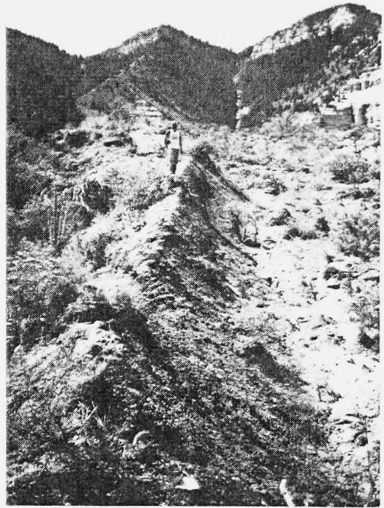
Figure 21. Twelve hundred foot long depositional levee along the eastern margin of the landslide. Refer to Figure 18 for location.
