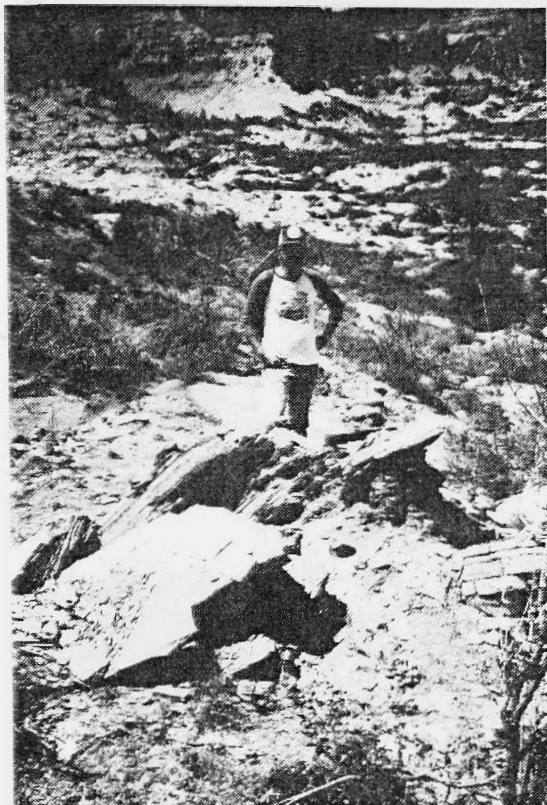
Figure 24. Highly fissile blocks of rock comprise the upper reaches of the landslide. Refer to Figure 23 for location.
