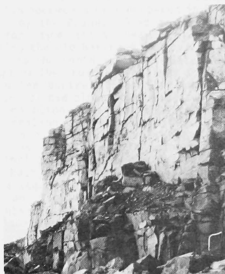
Figure 6. Top, southwestward view of the Rogers quarry on the west rim of North Table Mountain. Bottom, on the old quarry wall, notice how columnar jointing in the latite flow stabilizes the cut on the vertical face. Western Paving Construction Company plans to expand the old quarry eastward.
