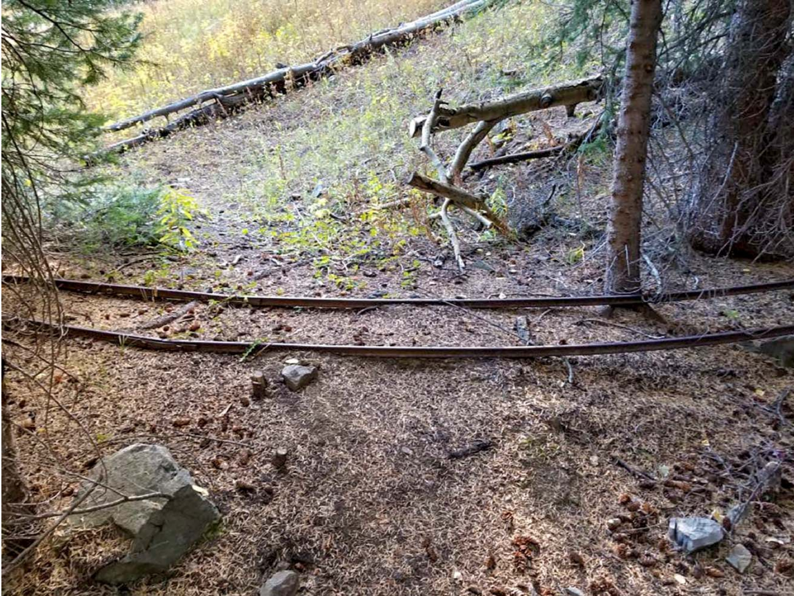
Figure D-9. Ore cart rails extending onto a mine dump from a collapsed adit. This feature was not identified in the AML-FS project or on the LiDAR.
