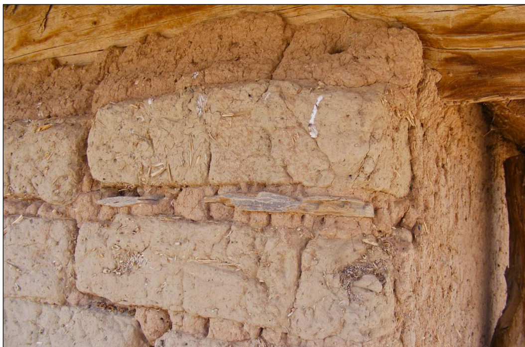
Figure 16. Detail of adobe bricks used to construct a modern storage shed on Cottonwood Mesa. The bricks and the mortar are made of mud and straw. The source of the clay is believed to be the Smoky Hill Member of the Mancos Shale. A couple of flat, lenticular rock fragments, possibly rippled calcarenite from the Juana Lopez Member or starved siltstone ripples from the Blue Hill Member, are incorporated into the wall mortar. [UTMX: 269,490, UTM Y: 4,294,528]
