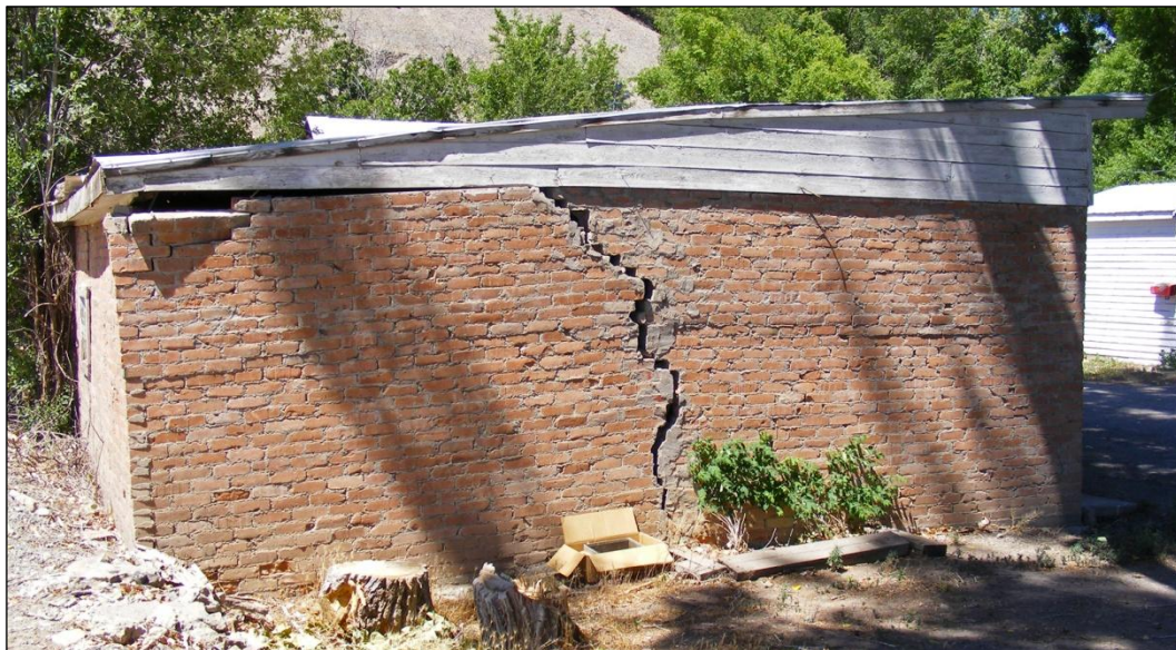
Figure 18. Garage damaged by collapsible soil and ground settlement in the town of Hotchkiss. This brick structure was built upon the alluvial fan ( Qf ) and mud fan deposit ( Qamf ) that underlies the main part of the town. A geotechnical well boring from nearby encountered 17 ft of potentially collapsible mud and gravelly mud deposits. Soil collapse issues are of concern for many western Colorado towns. [UTMX: 264,360, UTM Y: 4,298,379]
