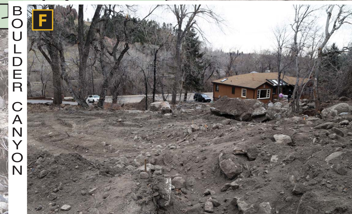
This debris fan along Boulder Canyon Road (Highway 119) impacted the rear of the home, causing half of the structure to move from its foundation. The fan also buried a portion of the parking lot. Location 40° 0'44.51"N, 105°17'50.02"W
