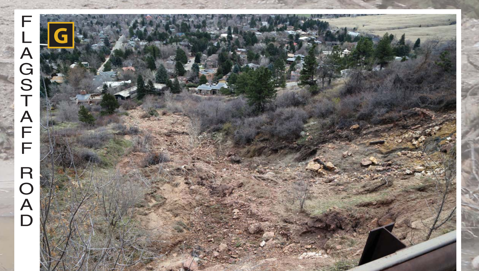
A mixture of boulders, soil, and plant debris threatened the neighborhood below and caused a portion of Flagstaff Road to collapse. Like many debris flows, it occupied a drainage where debris flows have occurred in the past and will likely affect these areas in the future. Location: 40° 0'11.07"N, 105°17'32.55"W
