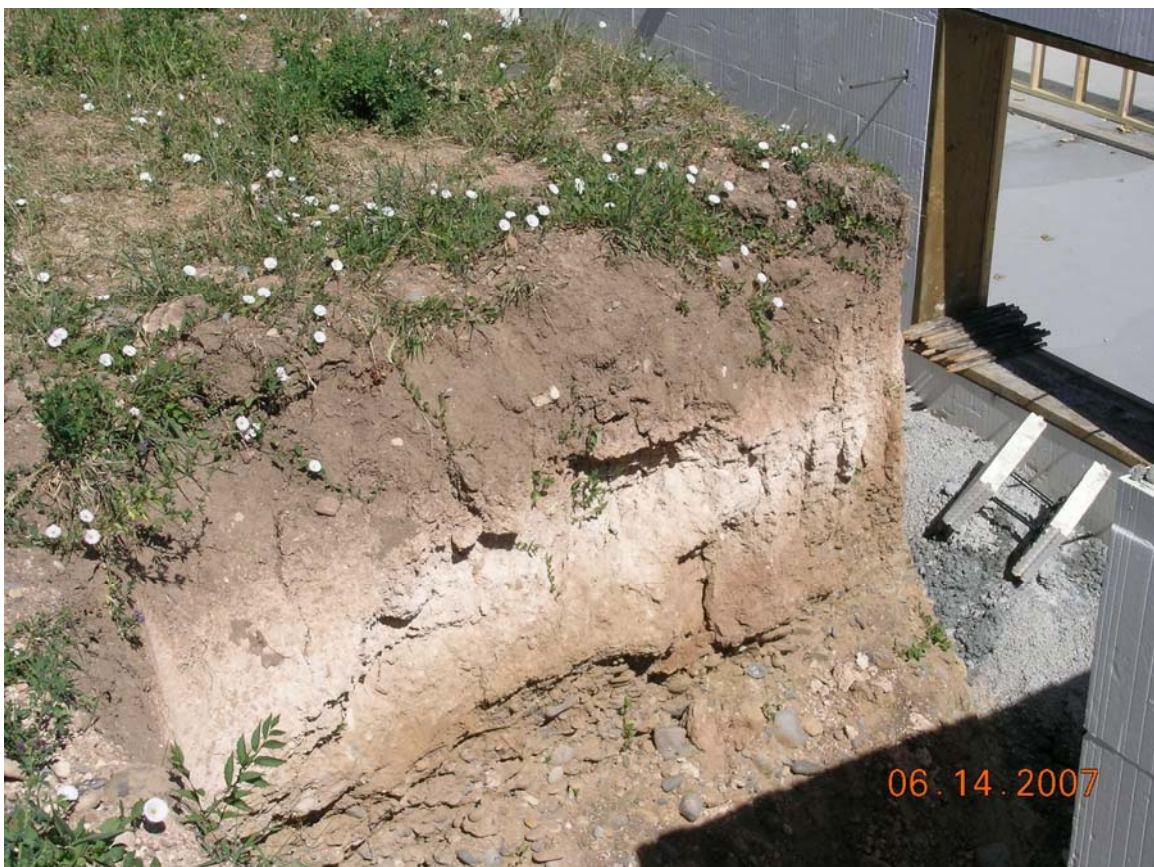
Figure 5. A foundation excavation on the \text{Qau}_4 terrace has exposed the fine-grained sediments that can overlie the gravels. Note the well-developed Bk/Bt soil horizons. The A horizon has been disturbed by previous agricultural use of this land. The Uncompahgre River gravels can be seen at the base of the excavation. [UTMX: 234916, UTM Y: 4277430].
