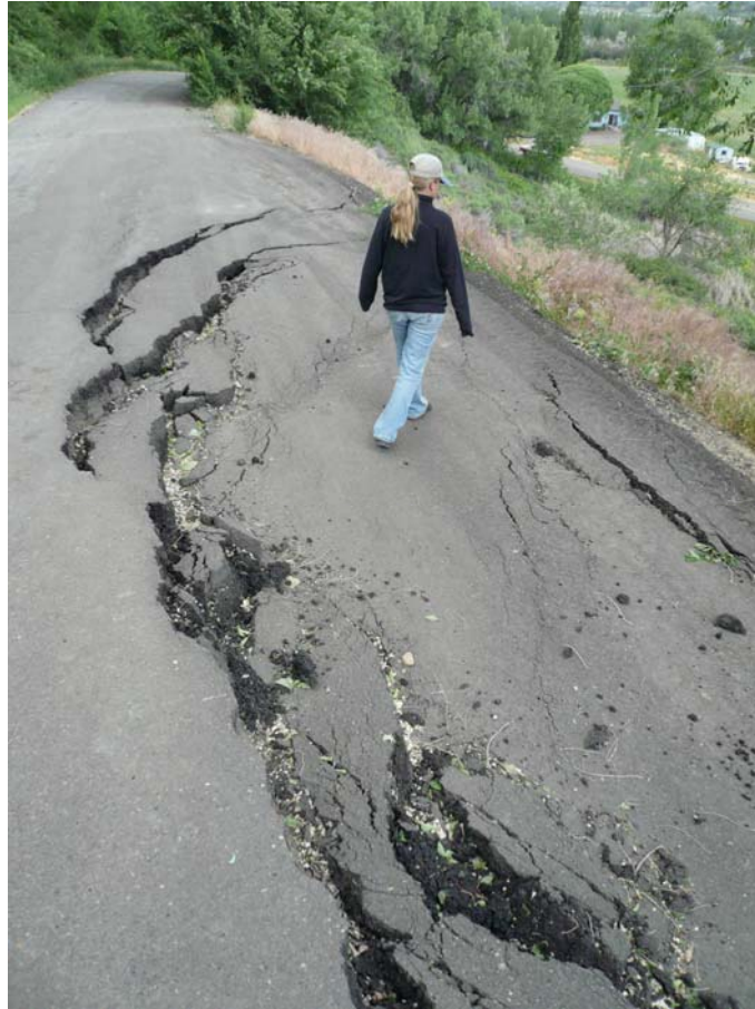
Figure 16. Damage to 1575 Road caused by a rotational landslide within the Mancos Shale. The road is now closed to vehicular traffic. [UTMX: 233542.8, UTM Y: 4288560.2]
