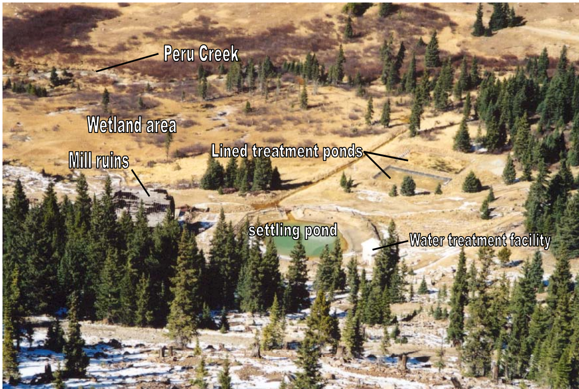
Figure 50. Pennsylvania Mill area, with inactive water treatment facility.
