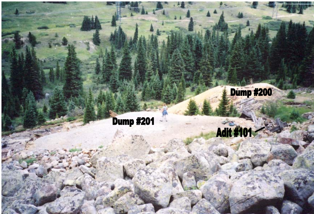
Figure 27. Adit #101 (collapsed portal timbers), dump #201, and dump #200.
