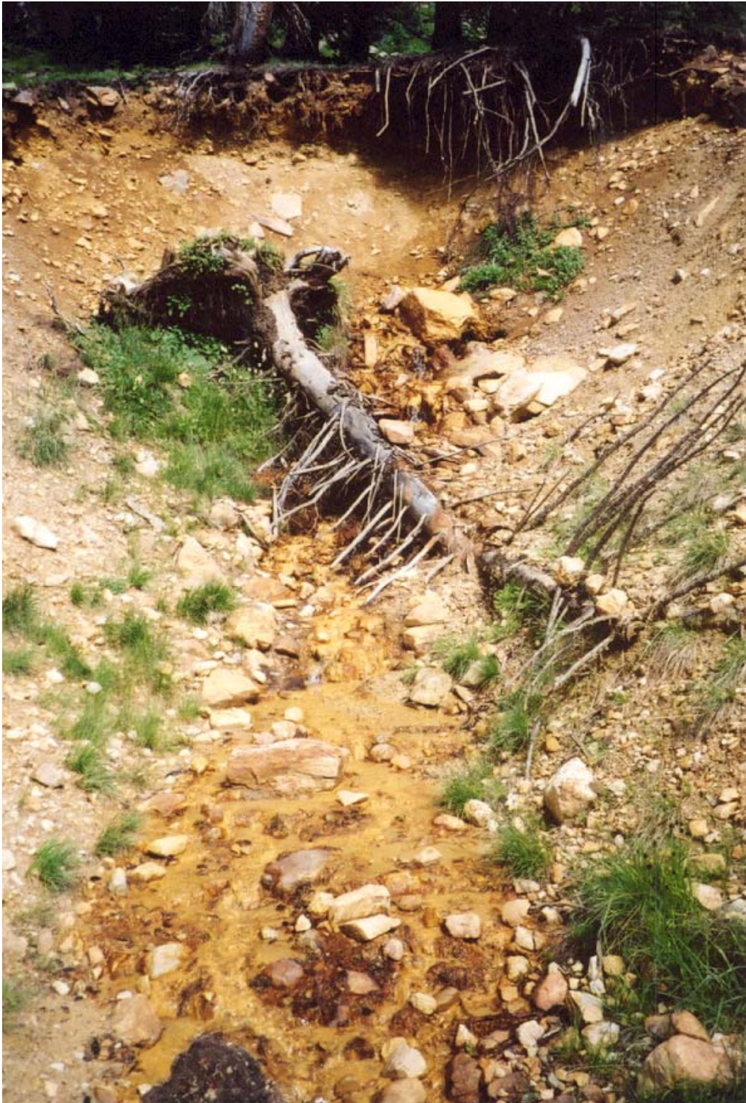
Figure 15. Effluent emerging from caved Delaware Tunnel (adit #106).
