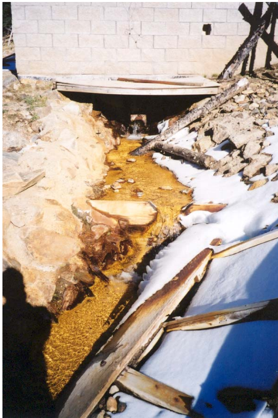
Figure 51. Effluent outlet from the inactive Pennsylvania Mine water treatment facility.
