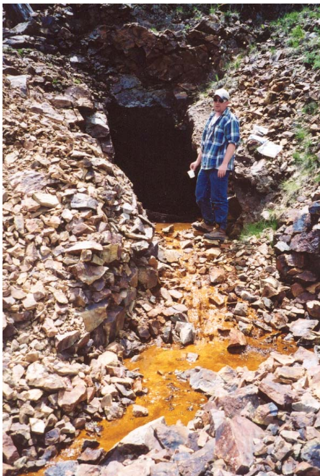
Figure 7. Adit #103 (Rich Ore Lode) showing effluent with orange precipitate.
