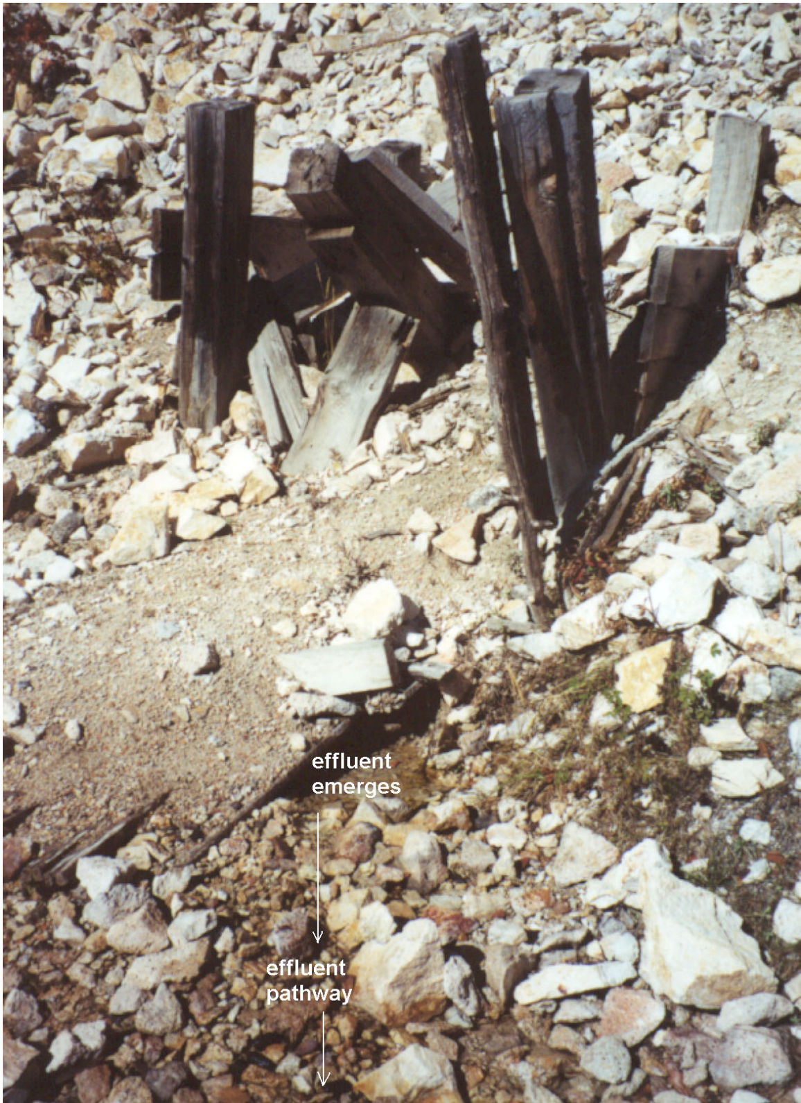
Figure 8. Effluent emerging from the caved Southern Cross portal.
