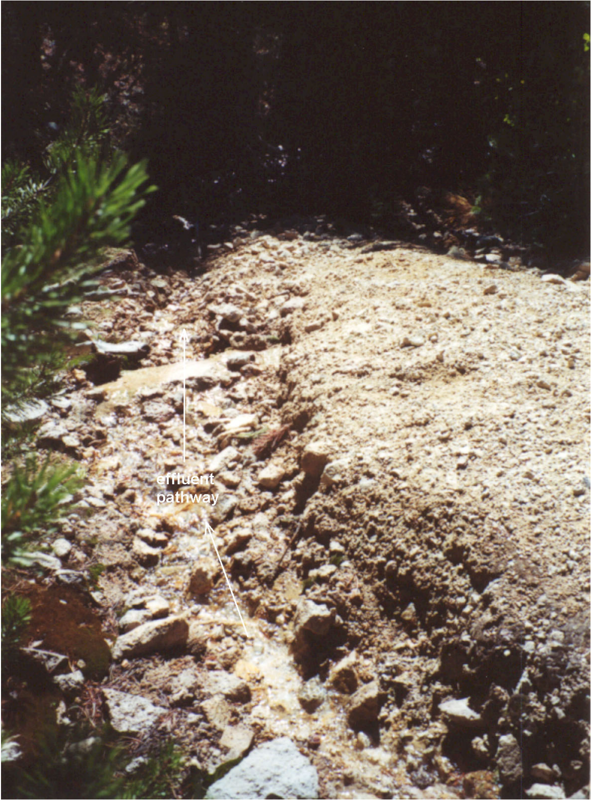
Figure 9. Gully and effluent on the eastern side of Southern Cross dump.
