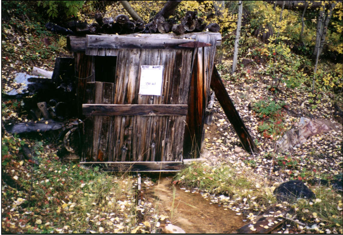
Figure 32. Enclosed portal and effluent at adit #102, New Dominion.
