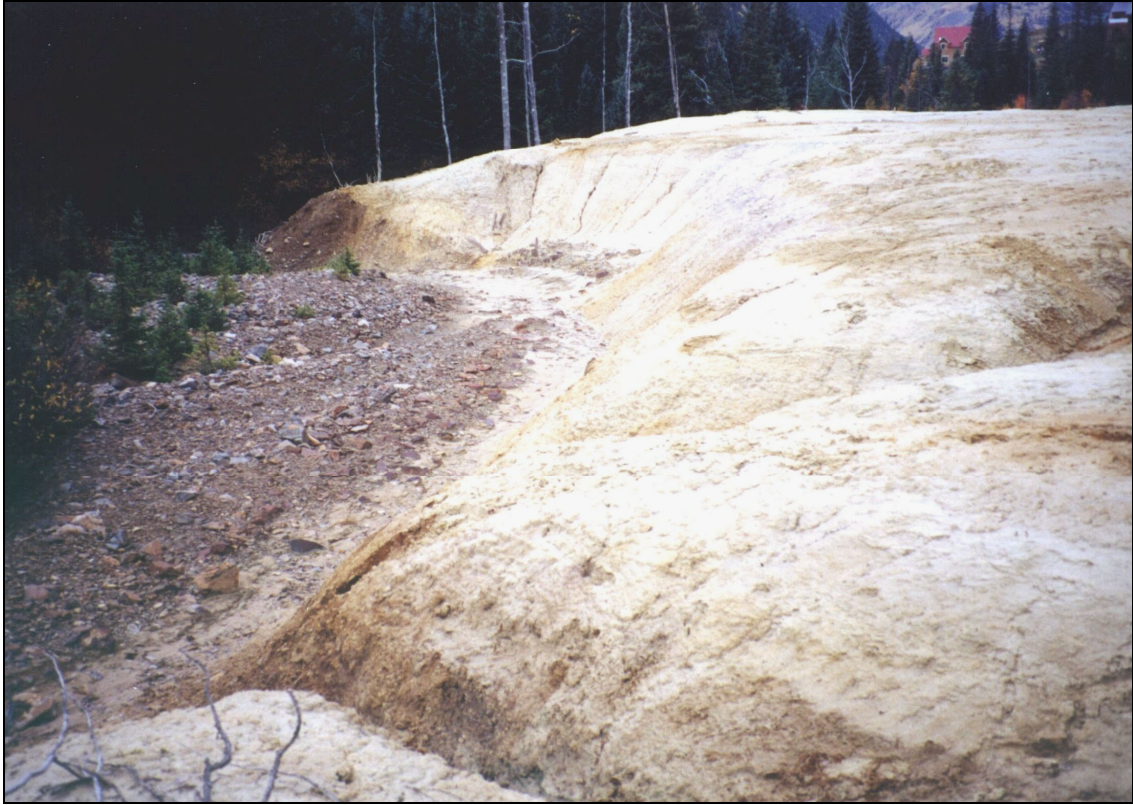
Figure 43. Thickest part of the Carbonero tailings pile, showing rills and gullies.
