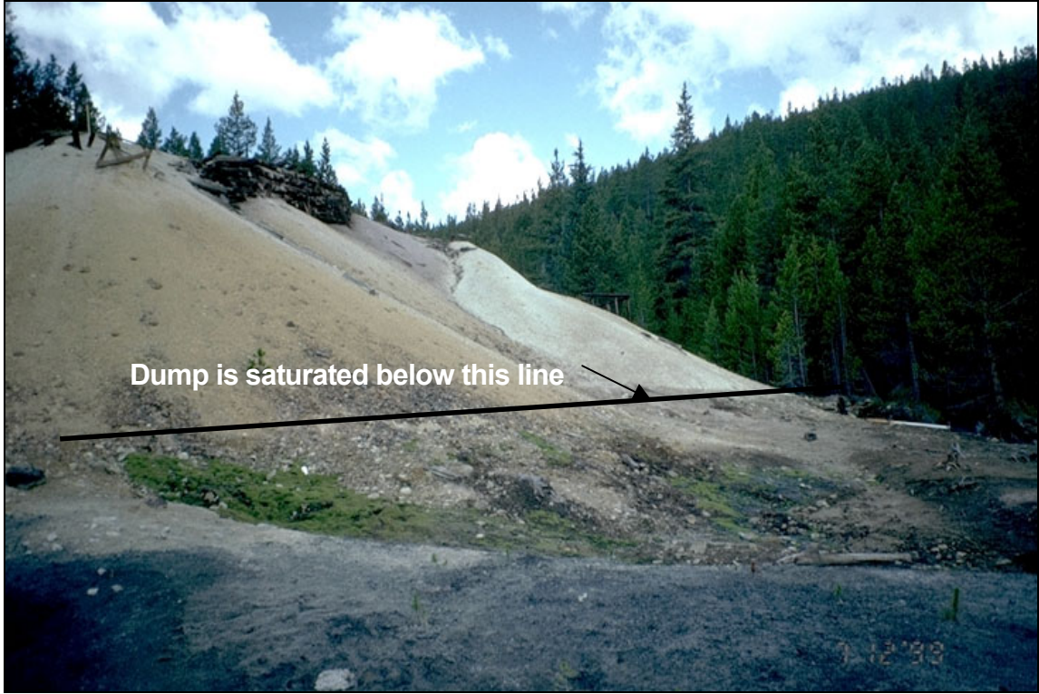
Figure 10. Photograph of seeps with vegetation and water saturation level in dump #200.
