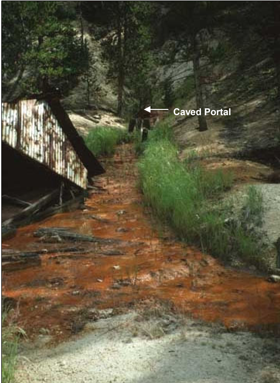
Figure 12. Photograph of caved adit #102 and effluent in 1996.
