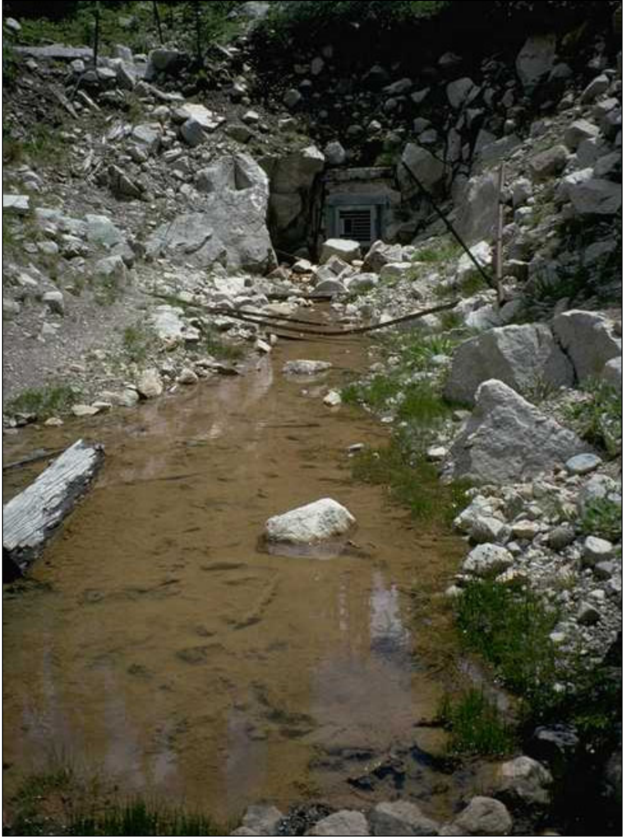
Figure 8. Effluent near the portal of the Stonewall Mine.
