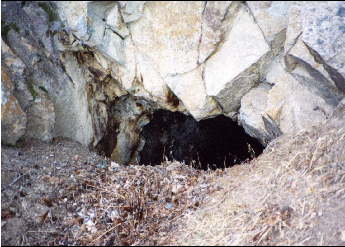
Figure 25. Nearly completely caved adit #100 in the “West Pomeroy Gulch” inventory area.
