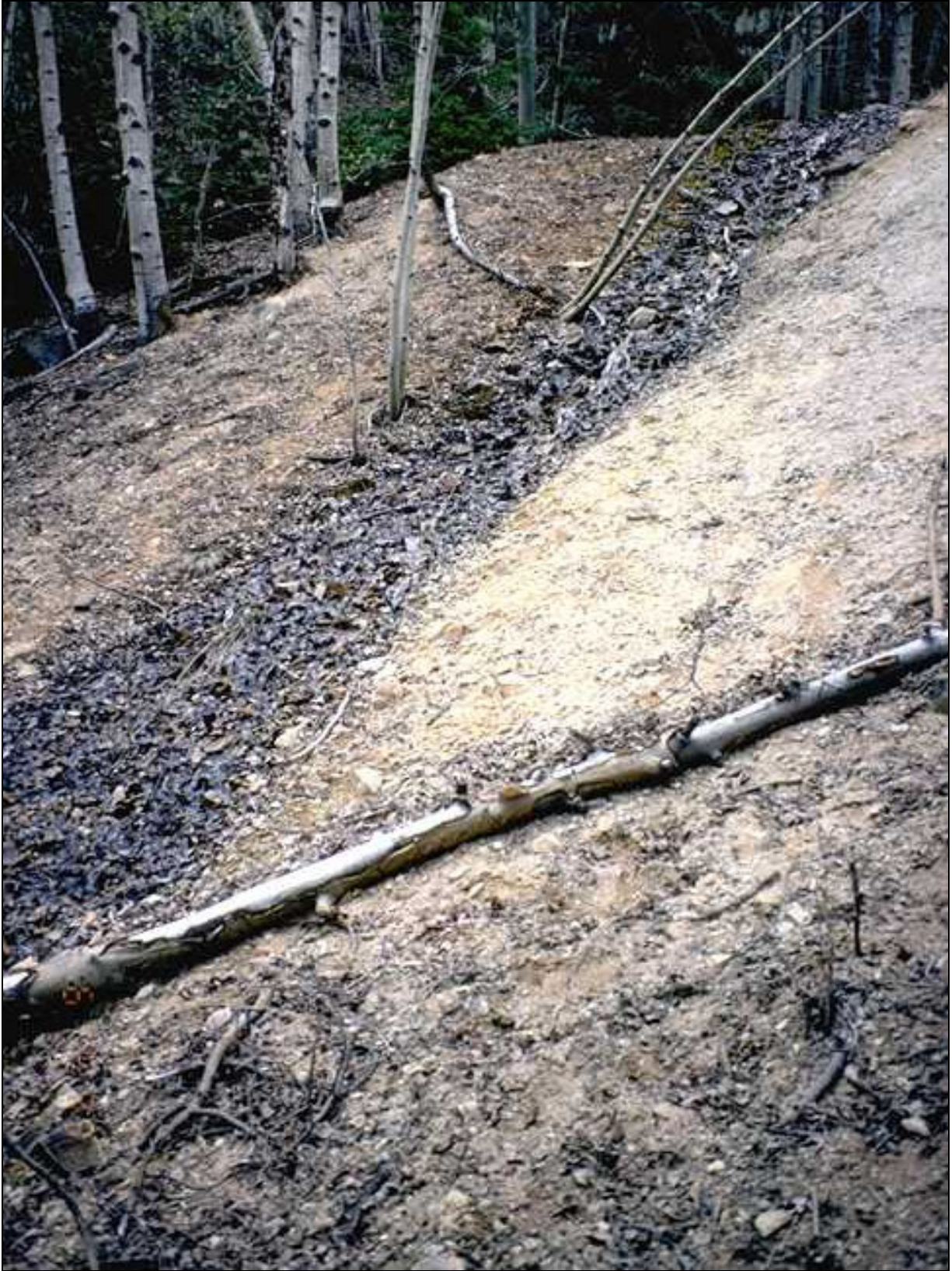
Figure 63. Water flowing down the face of dump #204 of the “Chalk Creek North” inventory area.
