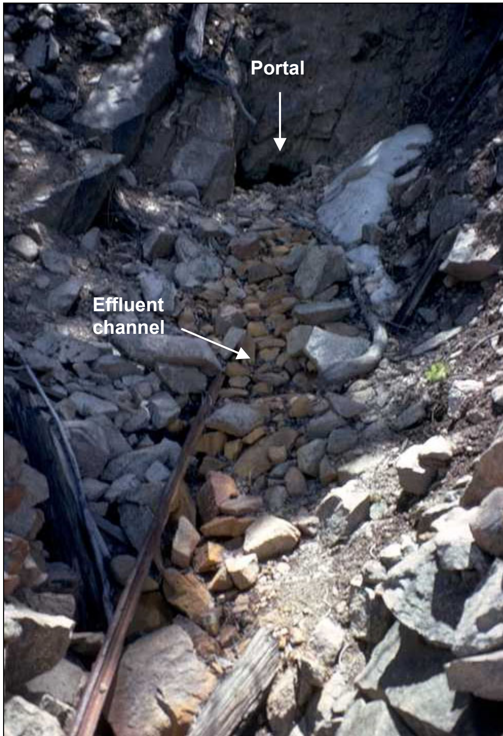
Figure 52. Mostly caved portal and iron-stained, dry effluent channel at adit #100, “Almost in St. Elmo area.
