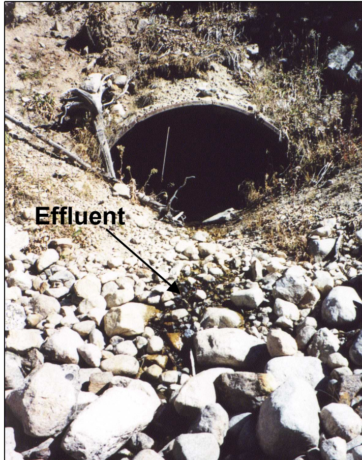
Figure 18. Culvert at the portal of adit #100.
