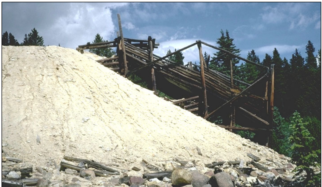
Figure 10. Rills and load-out chute on the Lienhart Mine dump.
