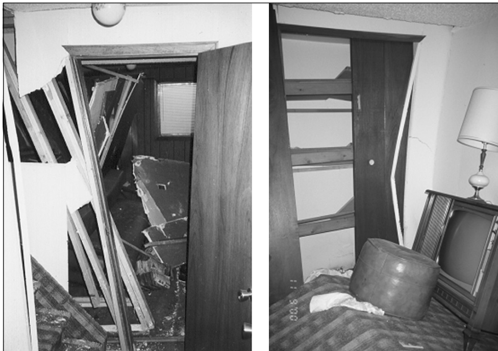
Figure 11. Ground movement caused this interior damage of a residence in the Hofstead Landslide in 1999. This home was condemned and later demolished. Photos courtesy of Hofstead Emergency Landslide Protection (HELP) Coalition and M. Squire.
