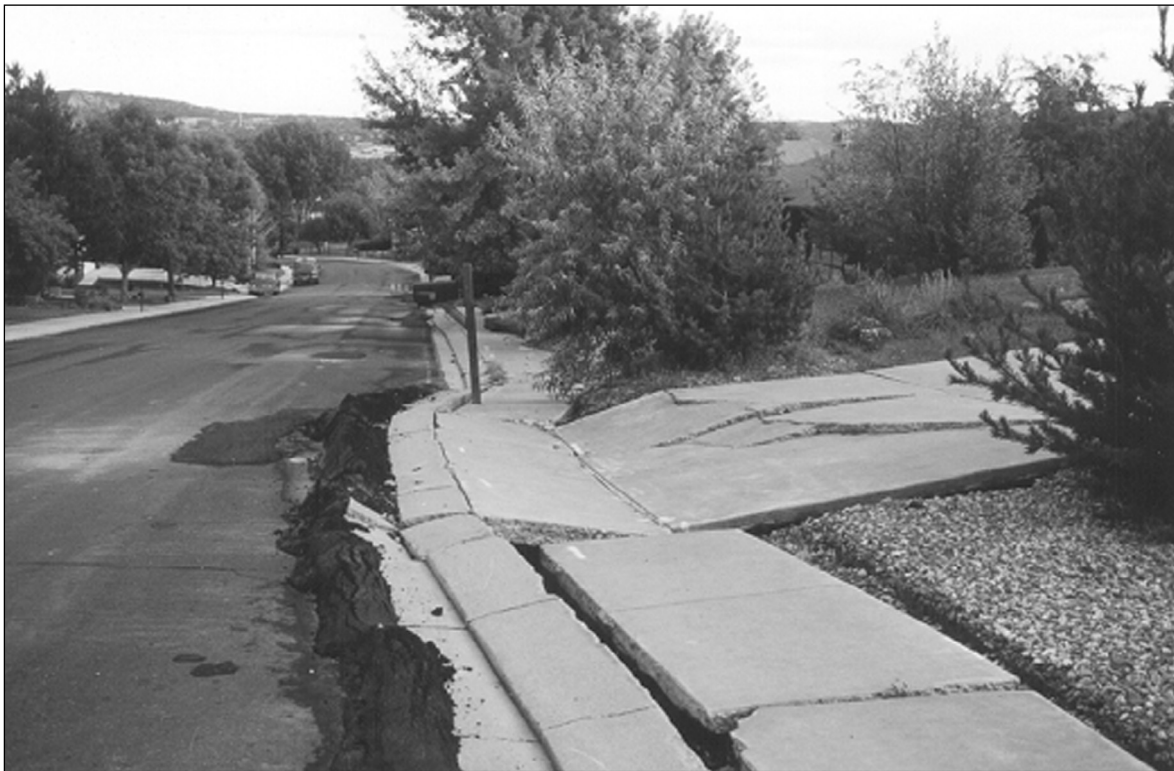
Figure 12. Damage to Hofstead Terrace roadway pavement, sidewalk, and driveway by lateral movement of landslide toe at Hofstead Landslide in 1999. Photo by J. White.
