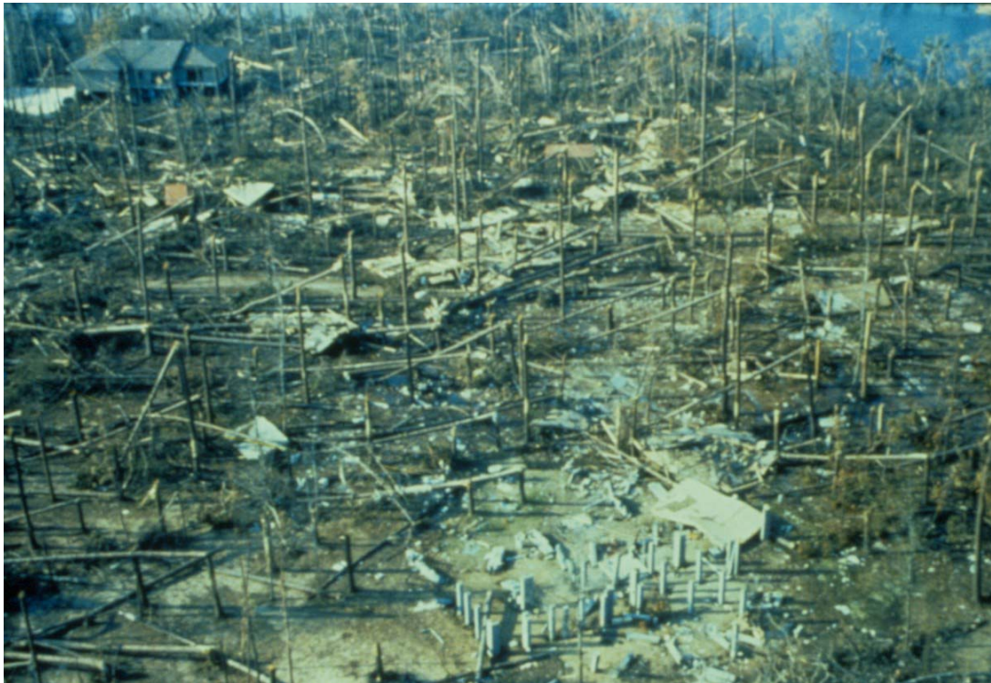
Destroyed area of Romain Retreat, on Bulls Bay, southern coast of South Carolina. Storm surge here during Hurricane Hugo was almost 20 feet. Forty-three homes were present before the storm. (photo from National Weather Service NOAA National Hurricane Center)
