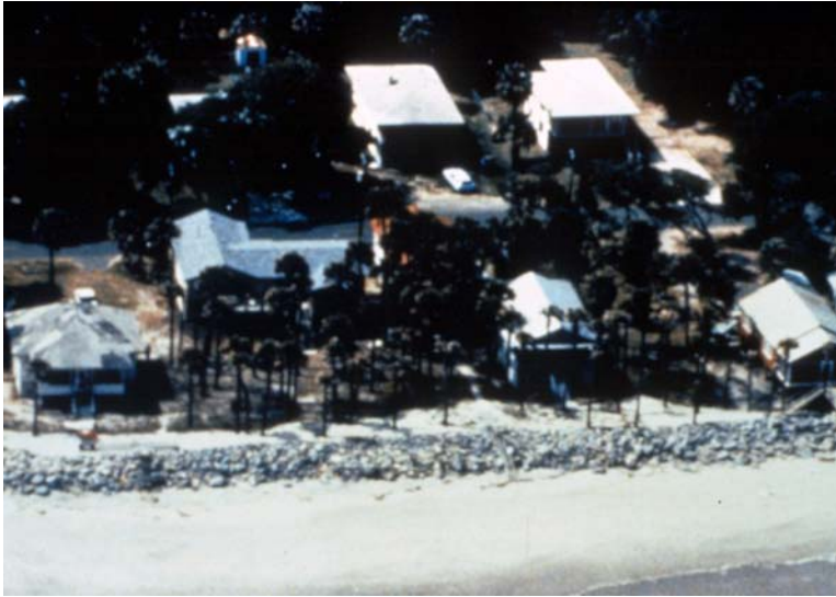
Folly Beach homes before Hurricane Hugo. Evidence of efforts to control beach erosion by engineering is revealed in the hard barrier of riprap rock facing the beach. The barrier was designed to protect homes by preventing wave erosion of the soft sand on which the houses are built.
