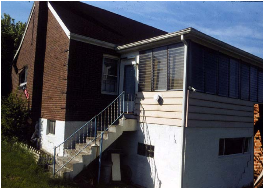
This brick home was declared a total loss to mine subsidence damage. Note that cracking occurs throughout the house, along the red brick side from cellar to roof (toward far left chinked with pink fiberglass insulation) to the concrete block foundation. Such homes are condemned and must be vacated. (photo by Edward Nuhfer)
