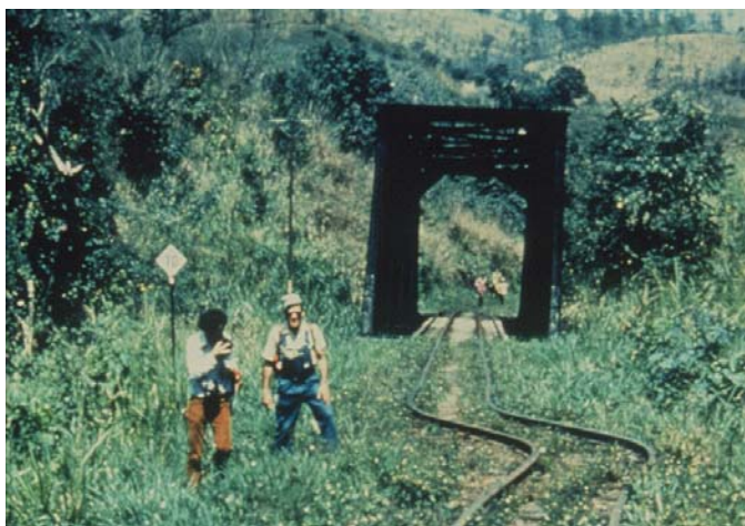
Railway in Guatemala offset by surface rupture. (photo from USGS photo library, Denver, CO)
