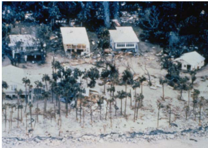
BELOW is the same housing area after Hurricane Hugo. The riprap rock barrier has been breached and nearly leveled by waves and storm surge.
