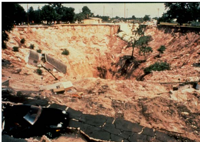
Sinkhole at Winter Park, Florida, engulfed homes, cars, recreational vehicles and part of a municipal swimming pool as the affected area expanded in early May of 1981. Damage developed over a period of a few hours, and within months the hole filled with water to form a new lake. A lowered water table caused by a dry season was thought to be the reason for failure during 1981. (photo by Florida Geological Survey)
