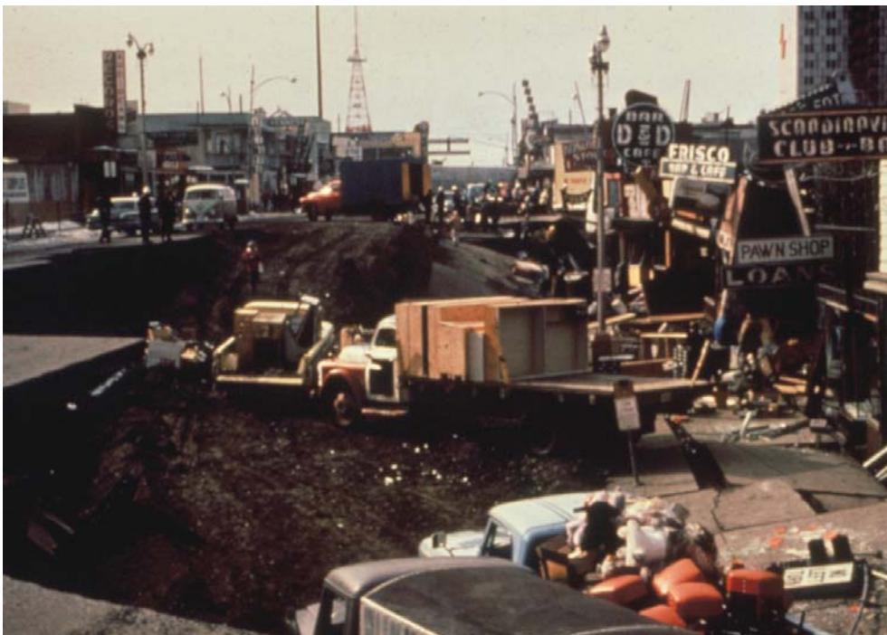
Compaction and settling of soft sediment formations beneath Anchorage, Alaska, led to destruction of the central part of town in the earthquake of 1964. Note the elevation difference between two sides of the street. (photo from USGS Photo Library, Denver, CO)
