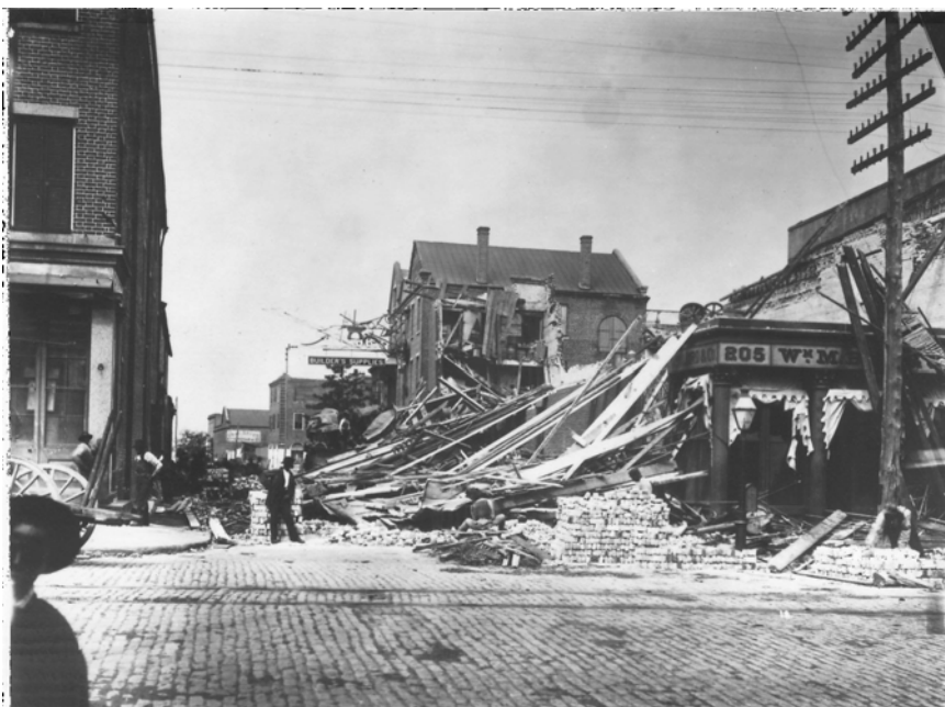
1886 Photograph of the Charleston, South Carolina, earthquake along East Bay Street. Because of infrequency with which major quakes occur away from plate boundaries, many property owners do not realize they are at risk and have no insurance against earthquake damage. (photo by J. K. Hillers; from USGS Photo Library, Denver, CO)
