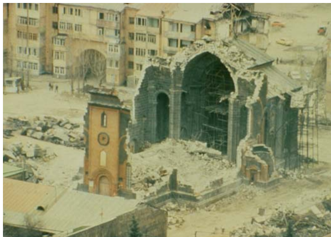
A casualty to ground shaking, an Armenian stone masonry church lies in ruins in the wake of the 1988 earthquake. High unsupported roofs in such public structures are responsible for large loss of life at a single site. (photo by C. J. Langer, USGS)
