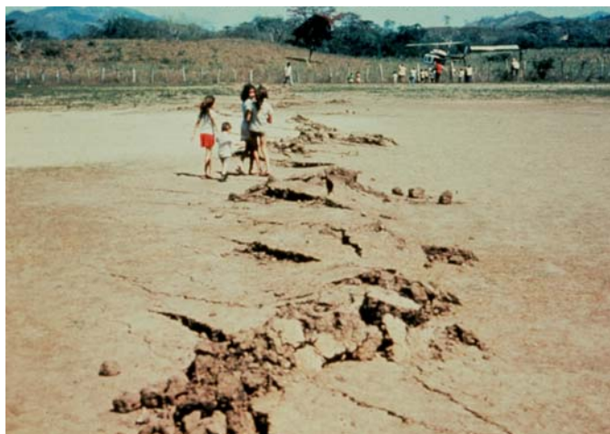
Ground cracking in Guatemala earthquake in 1976. (photo from USGS photo library, Denver, CO)
