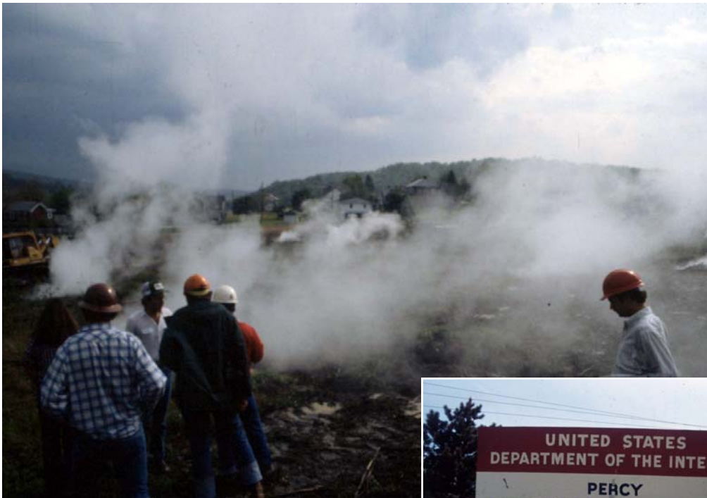
Underground fires in coal seams have been a major cause of subsidence. Workers at the Percy site in southern Pennsylvania encounter choking gases as they attempt to isolate the fire that otherwise would soon spread beneath homes in the background. (photos by Edward Nuhfer)
