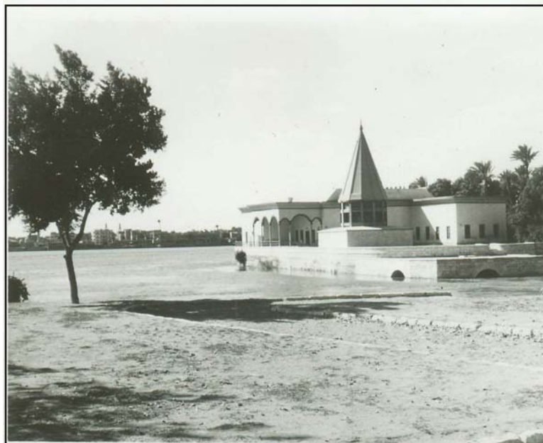
A nilometer on Roda Island near Cairo, Egypt. Several varieties existed; the earliest ones simply recorded the levels of the high water marks. These early stream gauging stations provide the longest hydrologic record in history. (photo by P. E. LaMoreaux)
