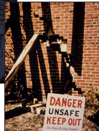
This brick home was declared a total loss to mine subsidence damage. Note that cracking occurs throughout the house, along the red brick side from cellar to roof (toward far left chinked with pink fiberglass insulation) to the concrete block foundation. Such homes are condemned and must be vacated. (photo by Edward Nuhfer)
