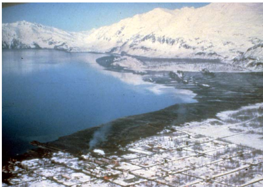
Aerial view of Valdez, Alaska, after tsunami damage. The wave was generated locally during the Alaska quake of 1964 when a huge block of land slid into the sea, carrying portions of the town with it. The landslide generated a huge wave that slammed into the waterfront within minutes and penetrated into two blocks of the town, producing 30 fatalities. (photo by U.S. Dept. of Interior, distributed by NOAA, Boulder, CO)
