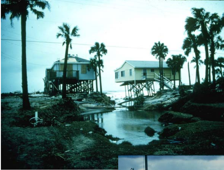
Sand movement affects homeowners in major coastal storms. LEFT - Scour produced in late stages of storm surge eroded the pilings of these homes almost to their bases on Folly Island, South Carolina.
