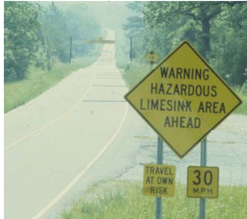
Sign warns motorists in the Dry Creek area of Shelby County, Alabama, about sinkholes that may appear suddenly in the highway built upon cavernous limestone. (photo by Paul Moser, Alabama Geological Survey)
