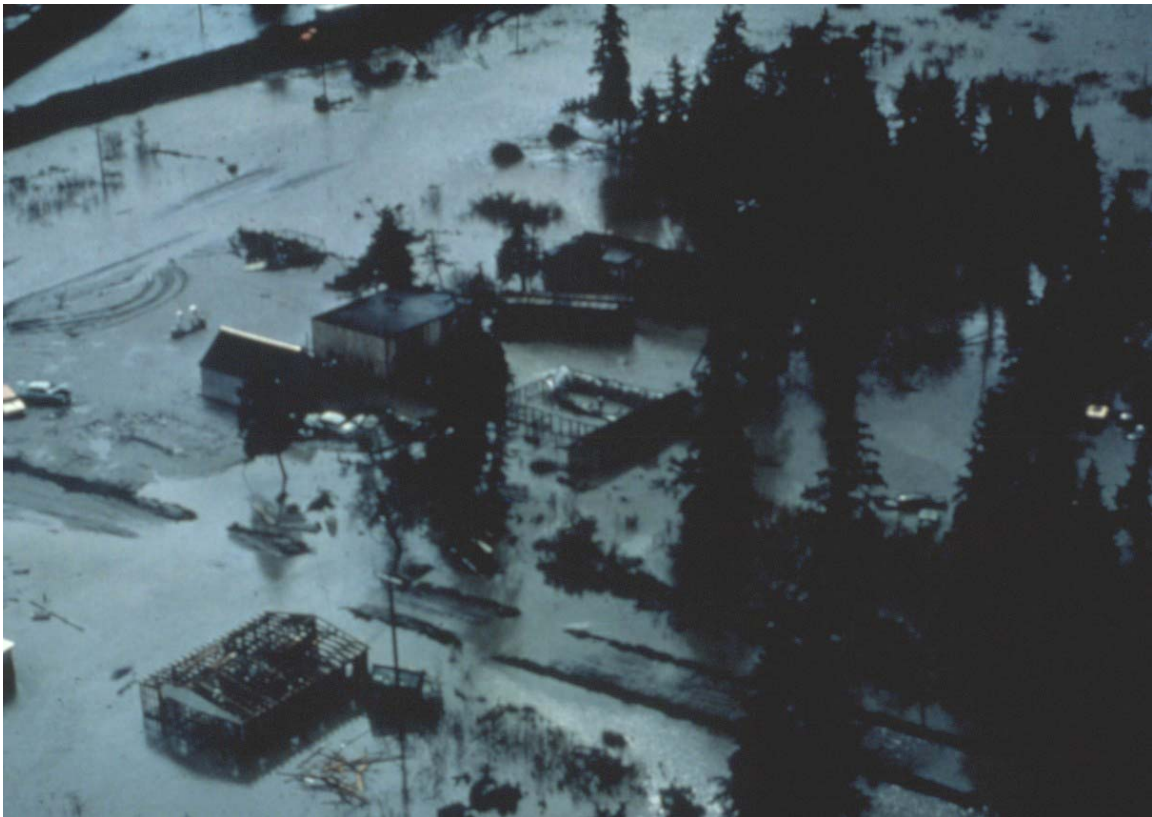
The town of Portage, along the coast of Alaska, was built on a block of land which subsided over 6 feet during the 1964 Alaskan earthquake. The town then flooded at every high tide. (photo from USGS Photo Library, Denver, CO)
