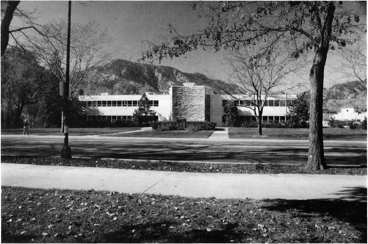
Figure 19. City of Boulder municipal building sited on the Boulder Creek flood plain less than 200 ft from the creek; location 6 on Figure 1.
