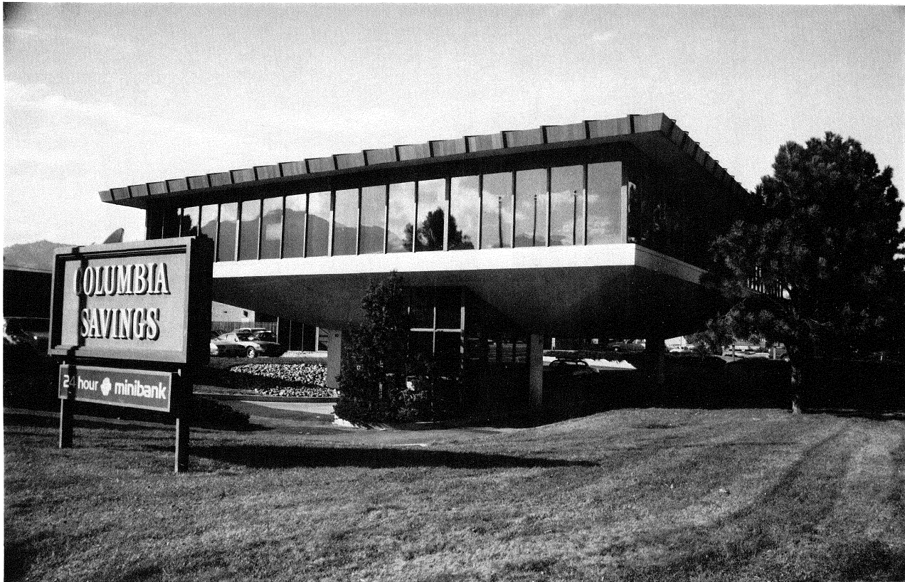
Figure 20. The Columbia Savings building, located on the flood plain of Boulder Creek, was designed with potential flood hazards in mind; location 7 on Figure 1.
