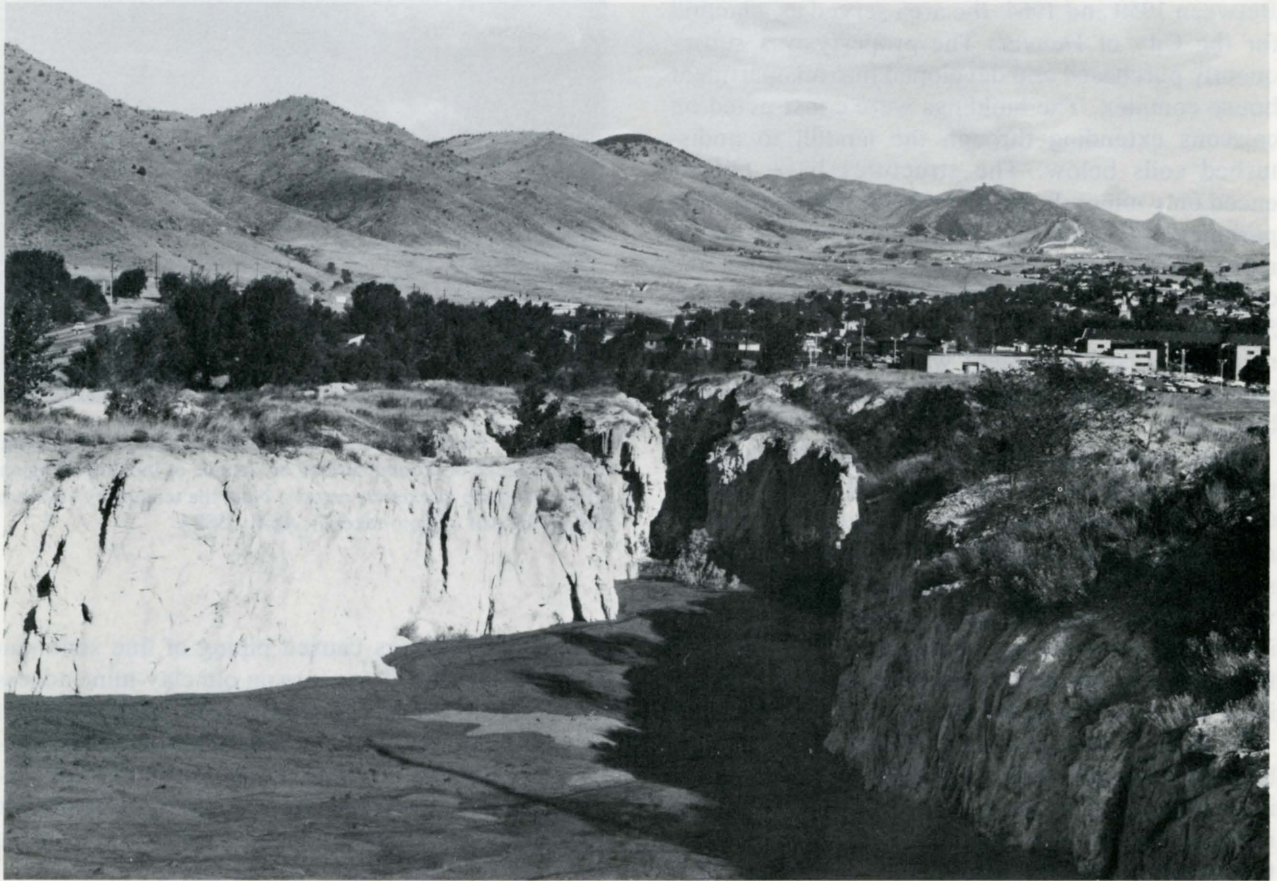
Figure 16. Fly ash slurry disposal as a stabilizing medium for reclamation of abandoned clay pits, Golden, Colorado. The fly ash is delivered by truck, in a wet mixture, over the 15 mi (24 km) distance from the Arapahoe Station of the Public Service Company of Colorado, in Denver. Approximately 3.5 \times 10^8 yd 3 ( 2.7 \times 10^8 m 3 ) are produced and delivered each week in a fleet of ten trucks. Mining of the vertically-bedded Laramie Formation clay strata has been going on since about 1876 by members of the Parfet family, who have been managing the fly ash disposal since 1979. Eventual reclamation of the clay pits is planned, with structural foundations designed to span the slurry fills, bearing on the Laramie interbeds (Photograph by Allen W. Hatheway, September 1980).
