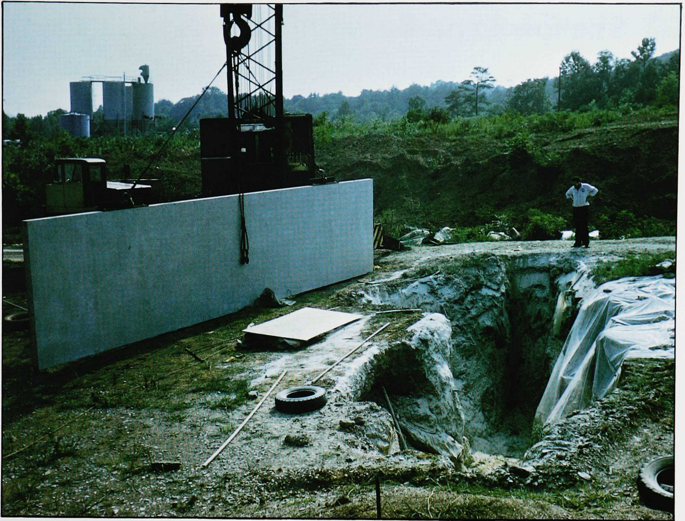
Cut-off wall to prevent ground-water dispersal of low-level waste
