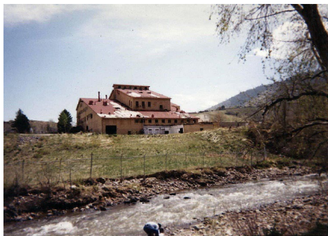
Fig. 59. Experimental Plant building shortly before demolition in 1997 and before construction of the Golden Kayak Run in 1998. View to southwest across Clear Creek, in foreground. Barbara Warden photo, used with permission.
