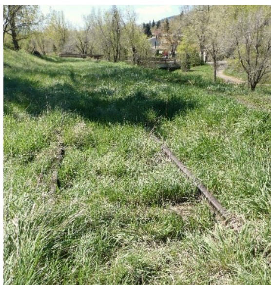
Fig. 96. Remaining tracks and rail bed along Tucker Gulch north of 1 st Street along Brickyard Branch on west side of North Table Mountain. View to south.
