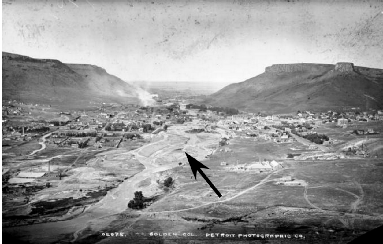
Fig. 51. 1882 view of Golden showing the braided channel (arrow) of Clear Creek. Smoke in background is from a smelter. View east. X9791, DPL WHC, used with permission.
