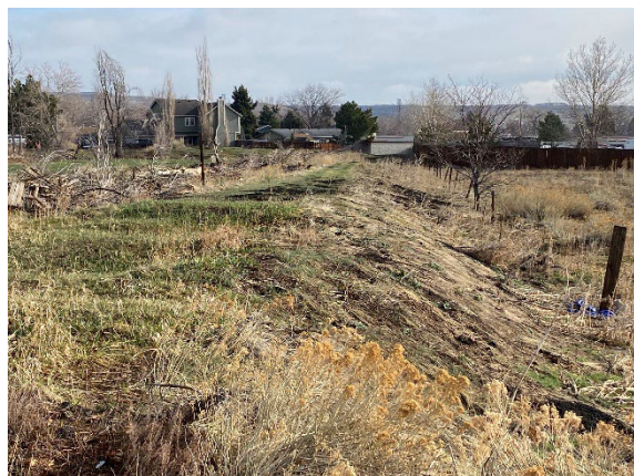
Fig. 99. Rail-bed embankments of the former Morrison Branch, east of the Golden Cemetery and Ulysses Street. Two weeks after taking this photograph, a development project removed the embankment. View to northeast in April 2021.
