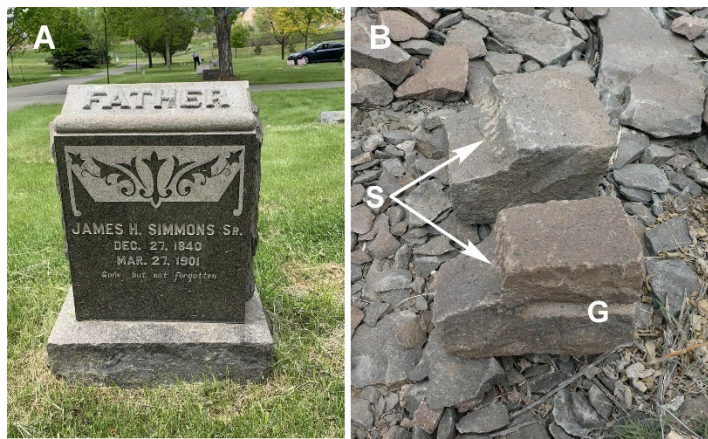
Fig. 91. A. Tombstone made of North Table Mountain basalt in the Golden Cemetery. B. Basalt paving stones at Tramway Quarry. Scoops (S, arrows) in stones accommodated streetcar rails. Horizontal groove (G) in bottom stone is from quarrying the rock.
