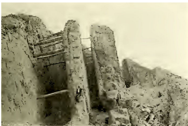
Fig. 78. Log “strain gauges” at the Hoyt Mine in 1901 with a man for scale. Photo from Geijsbeek (1901, p. 243).
