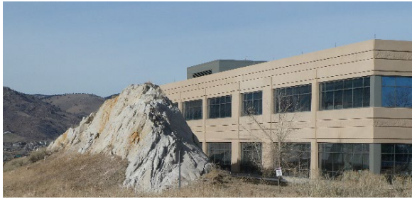
Fig. 25. "Fin" of white Laramie sandstone on the west side of the Jefferson County Laramie Building. View to northeast.
