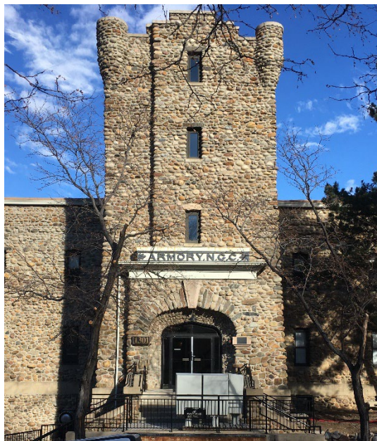
Fig. 50. Boulder walls of the Armory Building at 1301 Arapahoe Street are testimony to glacial floods that brought large rounded rocks down Clear Creek to Golden during the Ice Ages. View to east.
