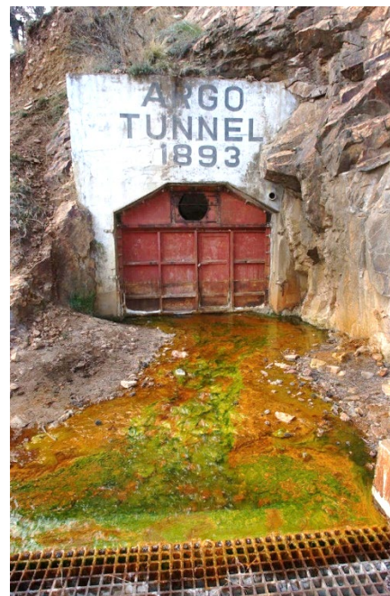
Fig. 58. Argo Tunnel portal in 2004 before remediation. Orange water is laden with heavy metals that, since 1998 have been removed before discharging to Clear Creek. 5401076.jpg, DPL WHC, used with permission.
