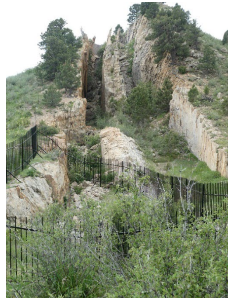
Fig. 100. In 2018, fences were installed around an abandoned vertical shaft at the former Tincup and South Golden fire-clay mines in south Golden after a near-tragic incident in 2017. View to south.
