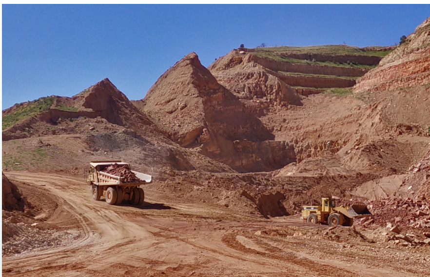
Pikeview quarry aggregate hauling, and conveyors (page 25), El Paso County. Photos Matt Morgan.
