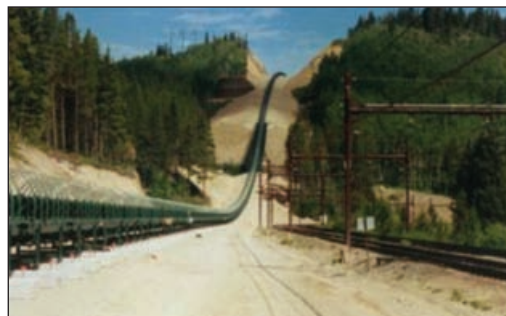
Figure 64. Ore is transferred beneath the continental divide to the mill in Grand County by means of a 15-mile long conveyor system. Once processed at the mill, the molybdenum-rich material, referred to as “concentrate,” is then transferred to the Freeport-McMoran plant in Fort Madison, Iowa, for refining into forms of molybdenum for sale. (Photo by Conveyor Service Corp.)
