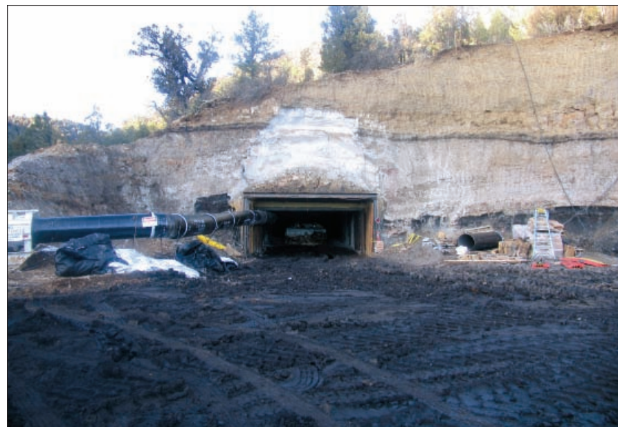
Figure 39. Construction activities at the new King II Mine, La Plata County. Shown are the main entry and ventilation systems. The coal bed is 6 to 7 ft thick, as shown in the cut slope face.
