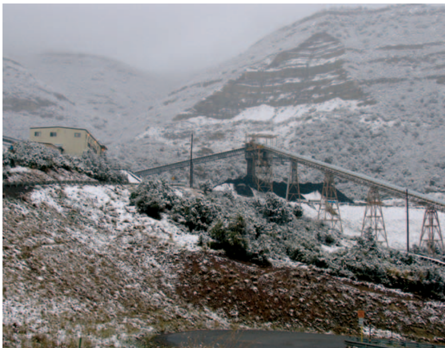
Figure 36. Conveyor system at the Bowie Resources mine complex in the North Fork Valley.
