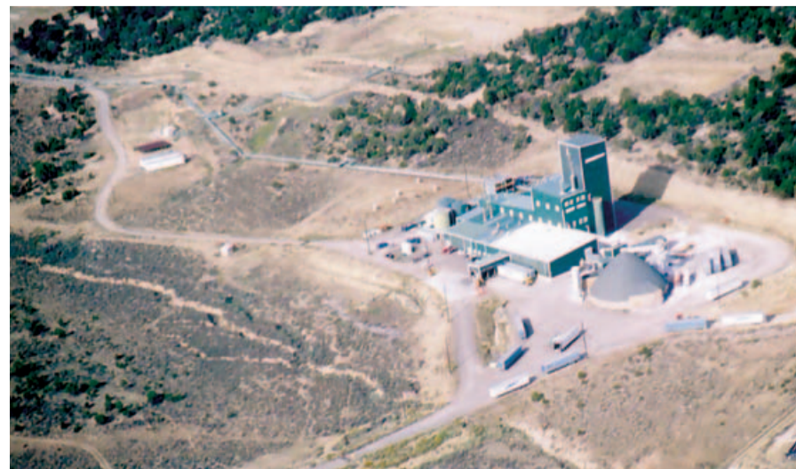
Figure 60. Aerial view of Natural Soda Inc.'s sodium bicarbonate plant in Rio Blanco County. Pipes that transport nahcolite-bearing solution from wells to the plant can be seen in the upper left. (Photo courtesy of Natural Soda, Inc.)
