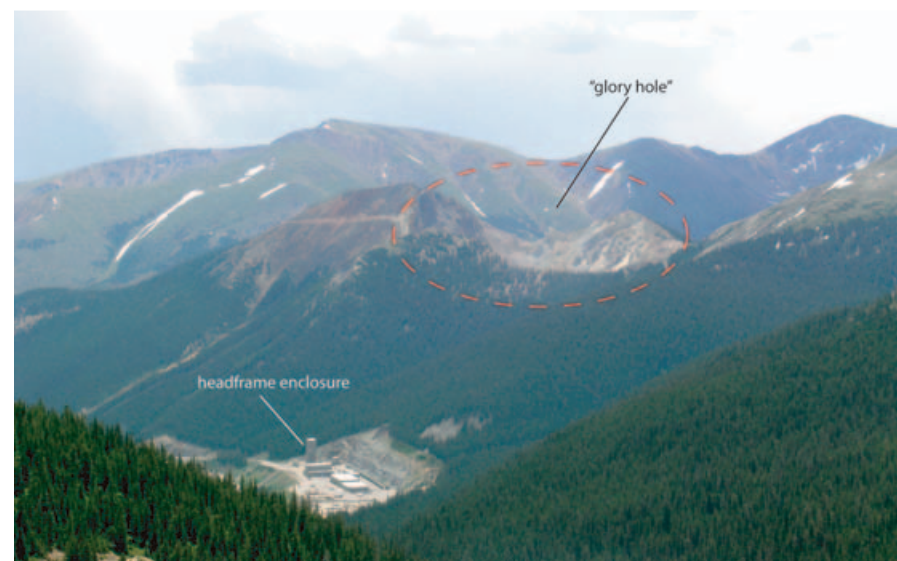
Figure 45. View of the Henderson Mine, Clear Creek County. The headframe for the main shaft is housed in the tall tower in the lower left part of the photo. Red Mountain rises behind the mine. The large “glory hole” (a sinkhole-like feature above the production area) is to the right of the summit of Red Mountain. (Photo by Jim Cappa, CGS.)
