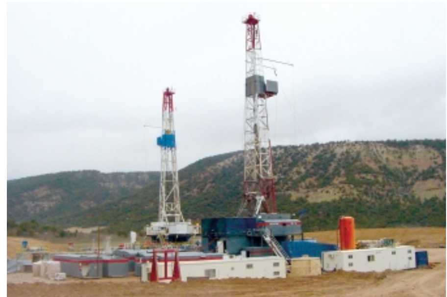
Figure 26: EnCana using multiple drill rigs on a single pad to drill and fracture stimulate wells in Garfield County; photograph courtesy Brian Macke, COGCC.
