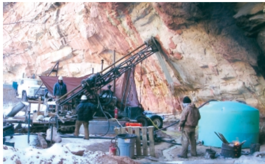
Figure 47. Core drilling hole 3CC-4 at a 30° angle up into cliff face of Wingate Sandstone at the Cashin copper deposit, Montrose County. Drill rig is a custom rig from Godbe Drilling LLC, Montrose, Colorado, modified to drill HQ-size up-holes specifically for this project; Photo by Jon Thorson; courtesy Constellation Copper, Inc.
