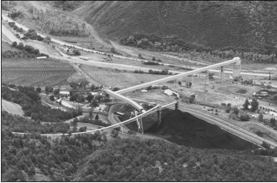
Figure 35. New surface loadout and conveyer system, Bowie No. 2 Mine.
