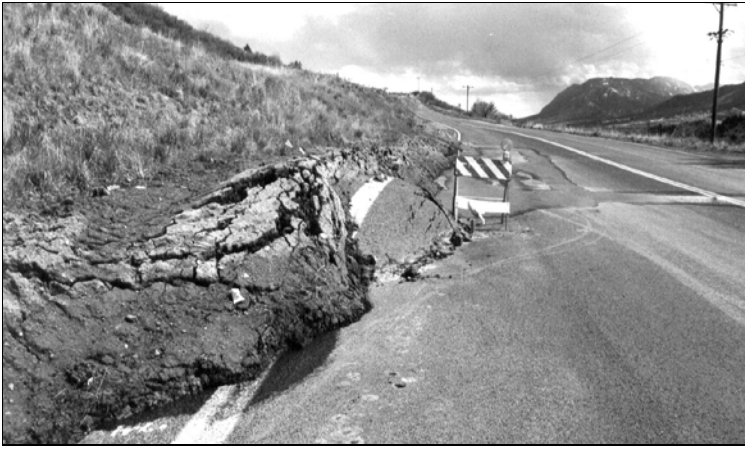
Landslide toe damages roadway (left) while the scarp damages bike path (right) in Colorado Springs. Photos by John Himmelreich.
