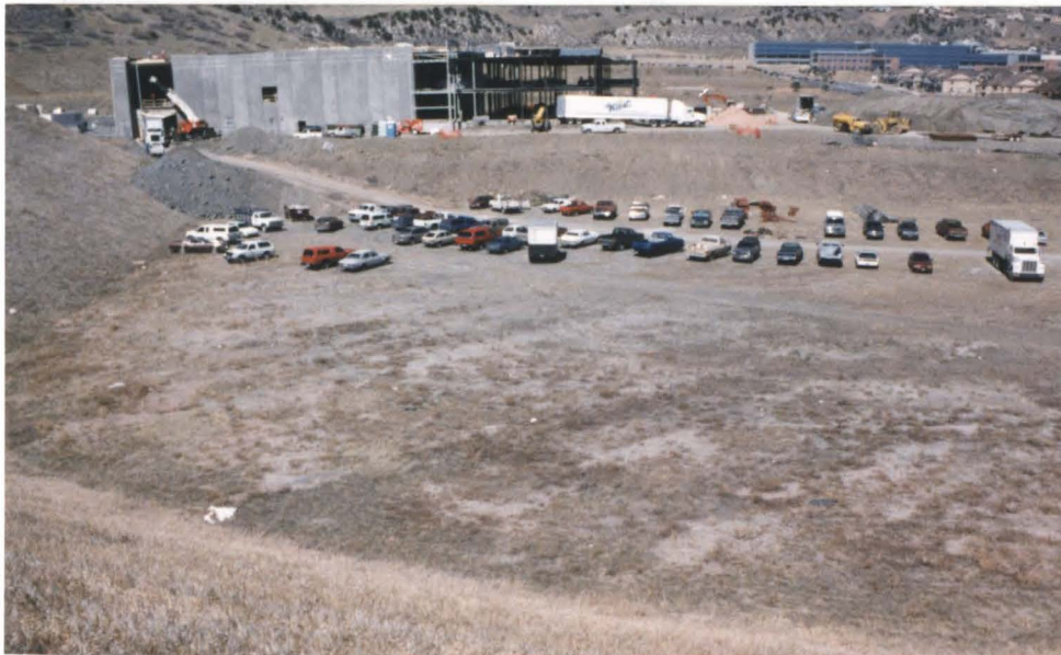
Several prominent linear heave features, which result from steeply dipping beds of expansive bedrock, cross a developed lot adjacent to an industrial development in Colorado Springs. All photos by John Himmelreich.
