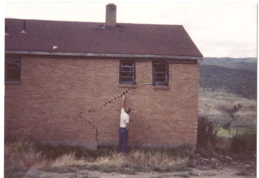
Soluble minerals in the Eagle Valley Evaporite formation are dissolved by groundwater. The resulting void sometimes causes subsidence at the surface. Subsidence (sink hole) resulted in this damage to a structure in Edwards, Colorado.
