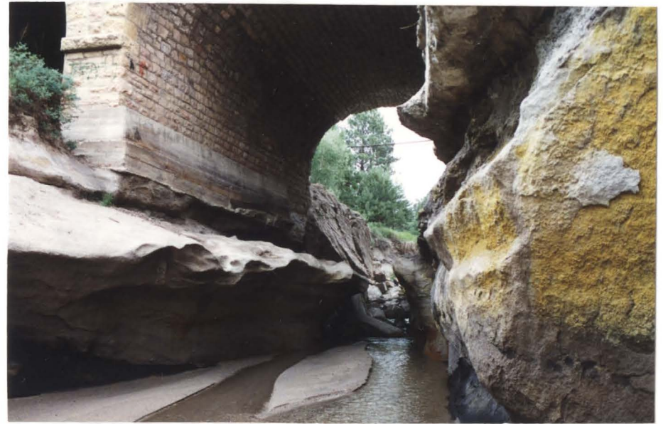
Even foundations resting on solid bedrock are subject to undercutting by the erosive effects of water.
