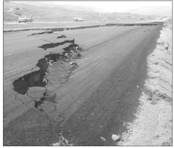
Slump encroaches on roadway and jeopardizes bike path (left). Photo by John Himmelreich. Landslide closes two lanes on Interstate 25 (right). Photo courtesy of the Pikes Peak Library District.
