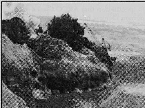
Figure 17a and b. Blasting operation in progress at Seneca Mine, Routt County. (Photos courtesy of Roy Karo, Seneca Coal Co.)
