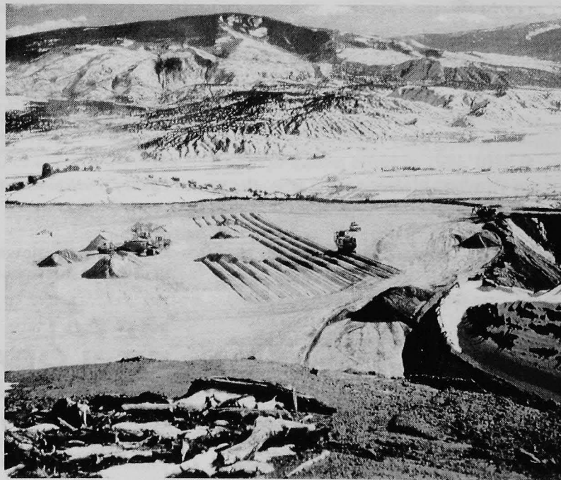
Figure 16. Eagle Gypsum mine, north of Gypsum, Eagle County. Note pavement profiler cutting furrows in gypsum bed. Loading facilities just to the left of photo center. Photo by J. Cappa, 1996.
