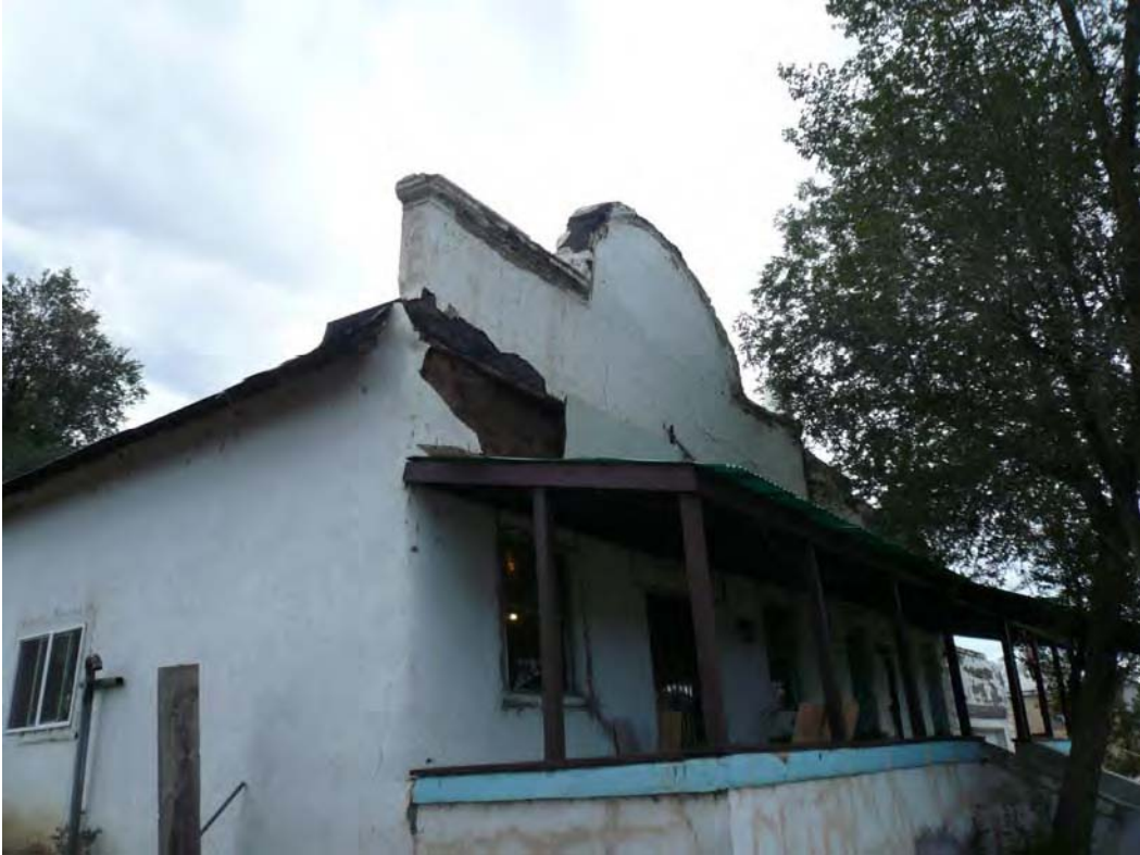
Figure 1. Highly damaged residence in Segundo where the façade has crumbled and pulled away from the main structure.
