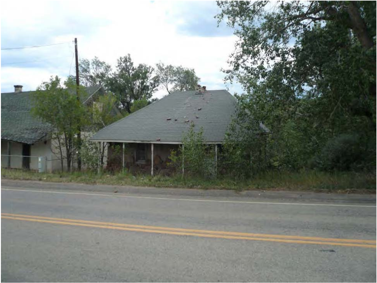
Figure 9. The earthquake toppled this chimney sending a few bricks onto State Highway 12. Segundo, CO.
