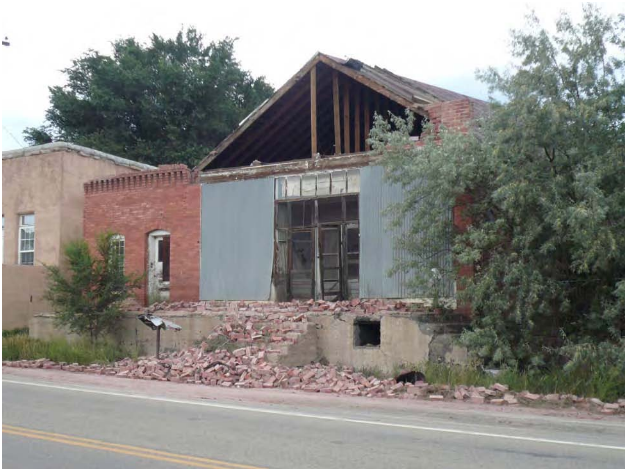
The front of this brick building collapsed, sending debris onto State Highway 12. Note the crushed mailbox. Segundo, CO.
